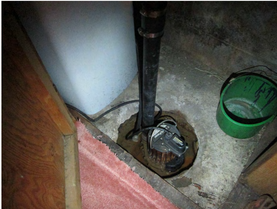
Photograph 14: View of the sump pump in the basement of Building A.
