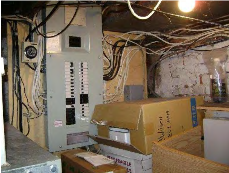
Combustibles stored near the electrical panel in the basement
