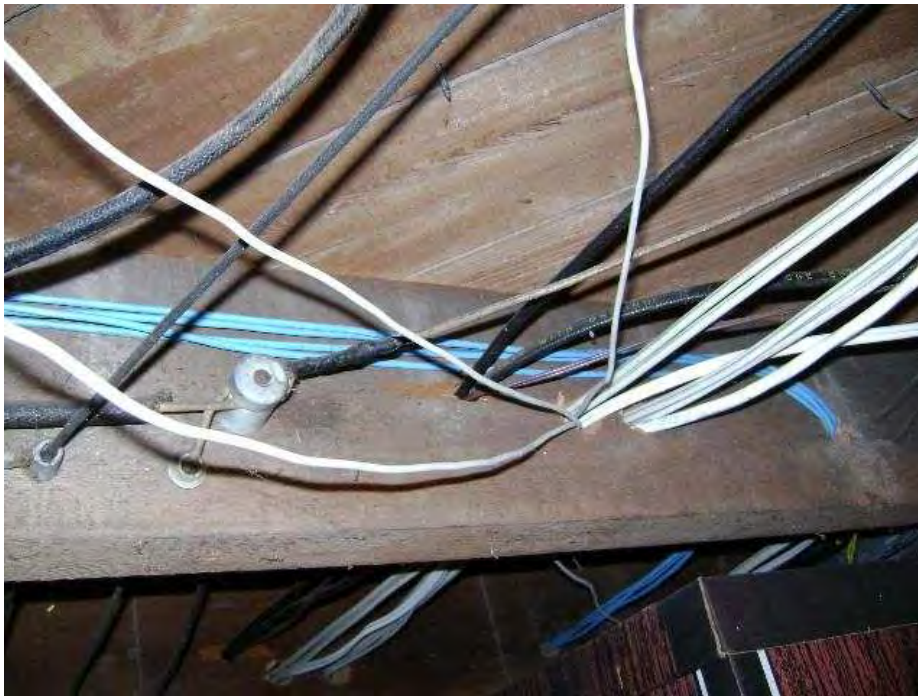
Typical electrical wiring in the building as shown below the basement's ceiling - Note the "knob and tube" wiring (Rec. Made).
