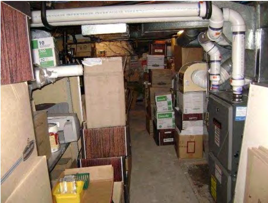
The basement showing stock of combustibles stored near the furnace
