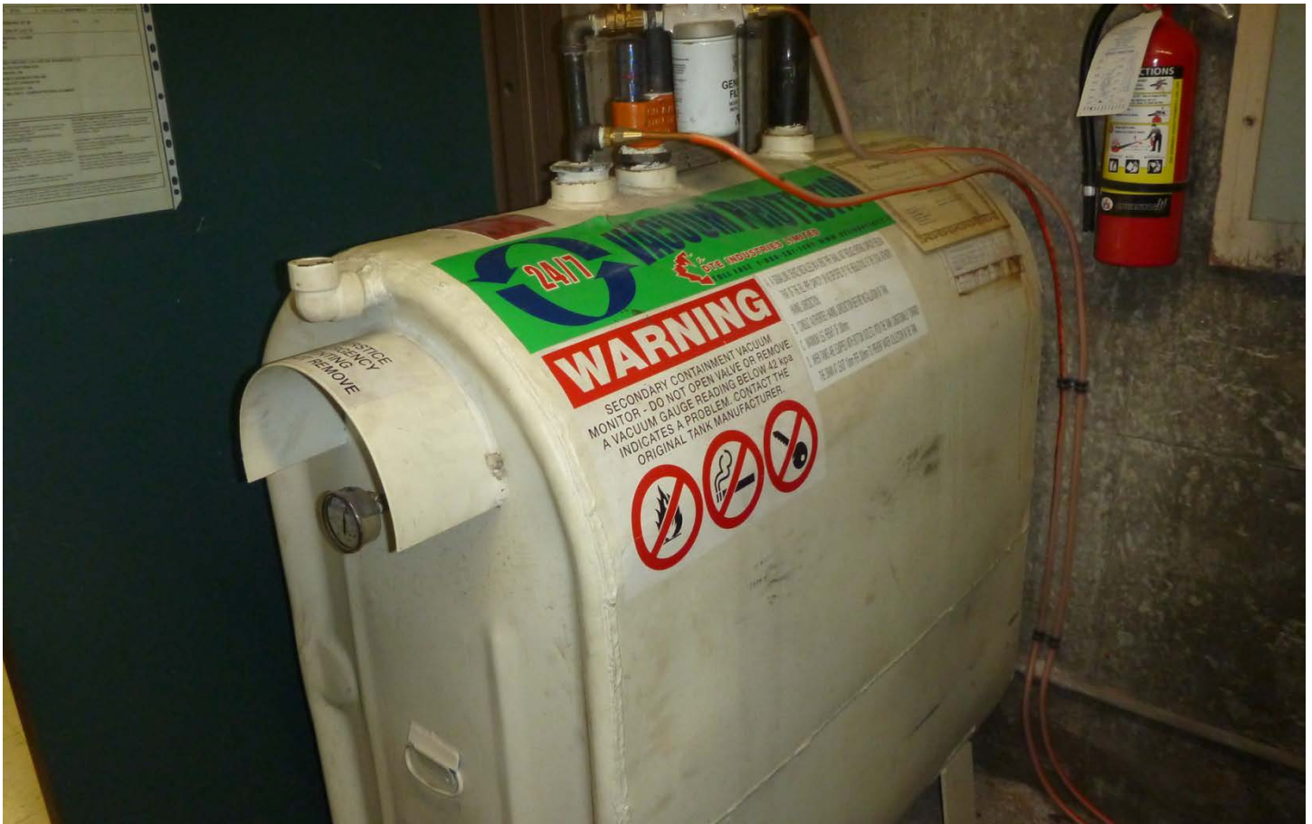
Photograph 5: View of an AST containing diesel fuel for a backup generator in the basement level of the Site building.
