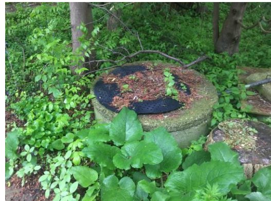
Picture 22: View of the abandoned domestic well located at the rear (east side) of Site Building A.
