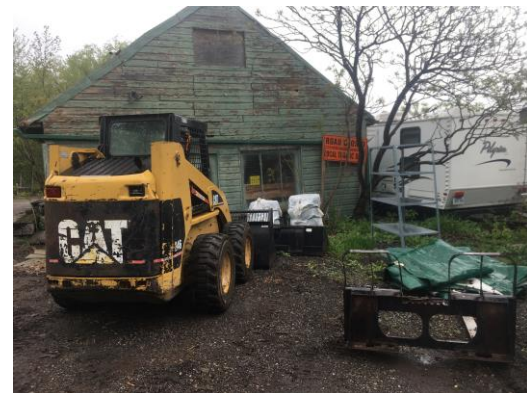
Picture 28: View of Site Building D on Parcel F facing south.
