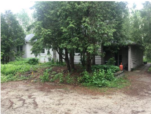
Picture 21: View of the front of Site Building A off of Ninth Line facing west.
