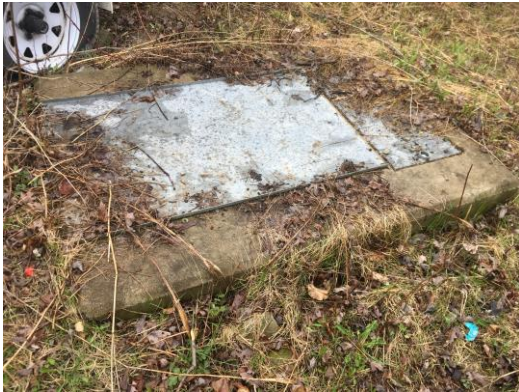
Picture 19: View of the underground hydro located near the cell tower on Parcel E.
