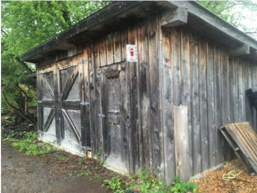
Picture 27: View of Site Building E facing north.
