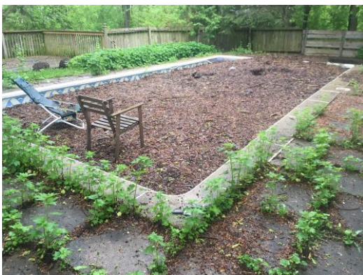
Picture 23: View of the swimming pool at the rear (east side) of Site Building A.
