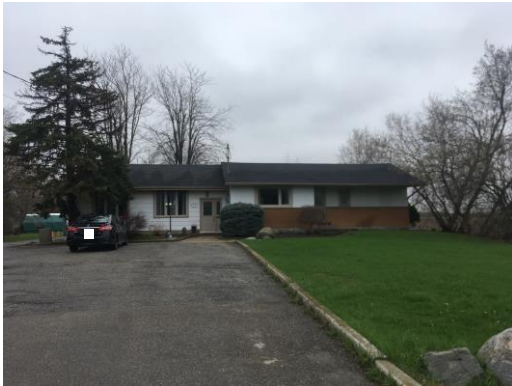
Picture 1: View of the front of the residential dwelling on Parcel E. Overhead hydro cables can be seen leading to the roof of the Site Building H.
