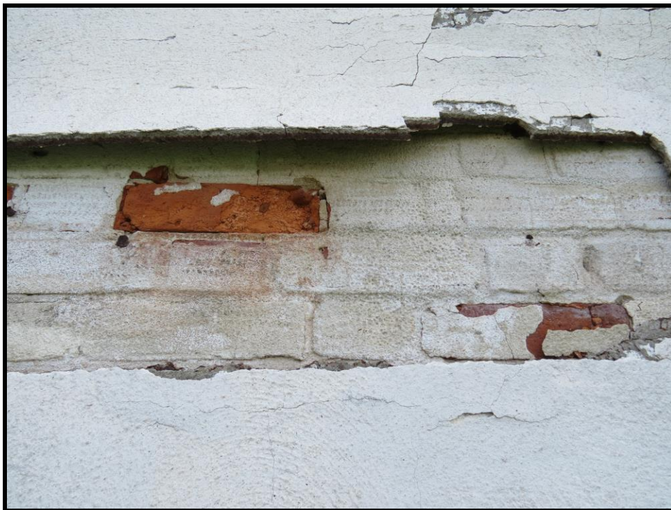
Image 29: Detail of stucco cladding over red brick structure (Photo taken on June 13, 2018; Facing South)
