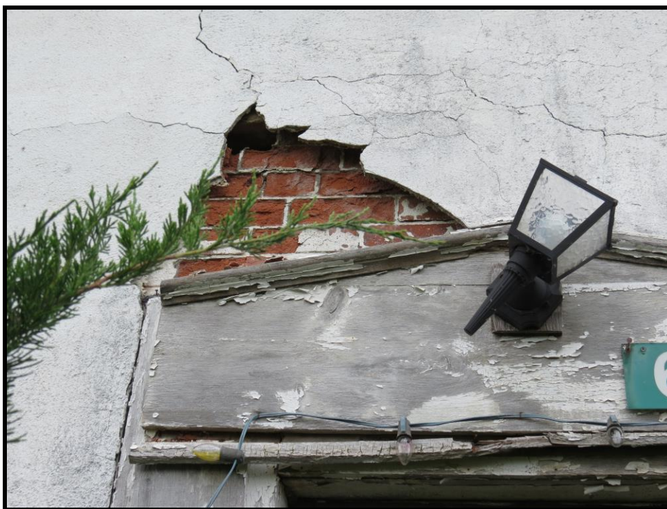
Image 10: Detail of stucco cladding over red brick structure (Photo taken on June 13, 2018; Facing West)
