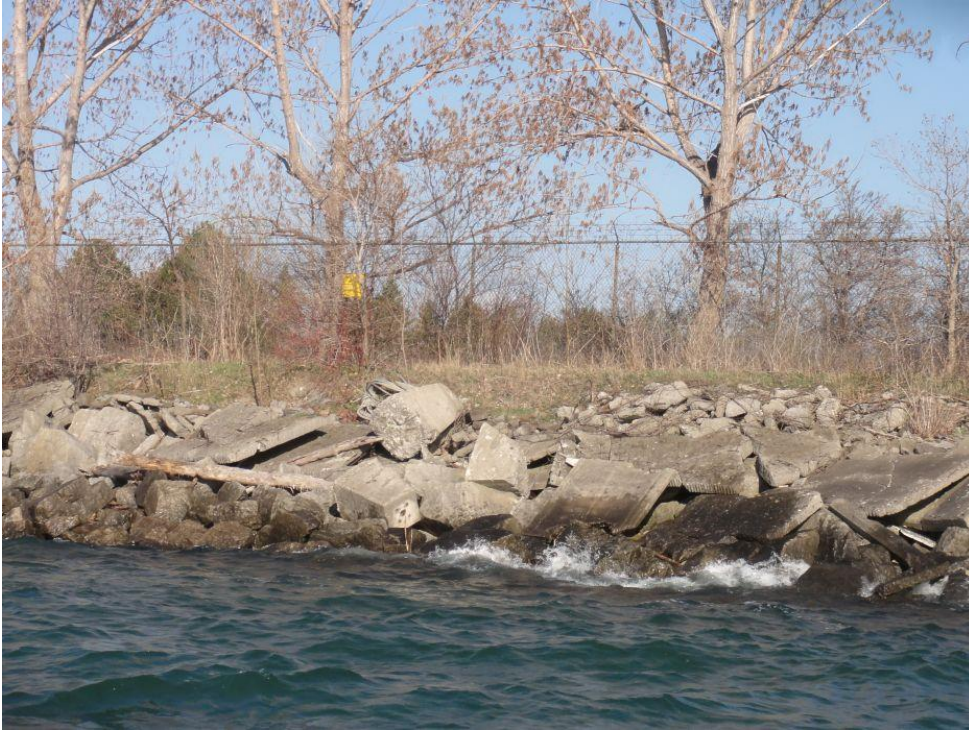
Figure 2.30: Example of concrete rubble on revetment at westerly portion of Outer Shore
