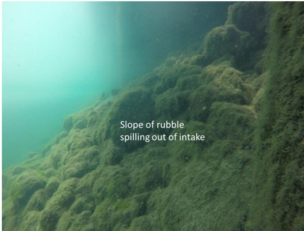
Figure 2.74: Rubble slope spilling out of intake at Pumphouse 3
