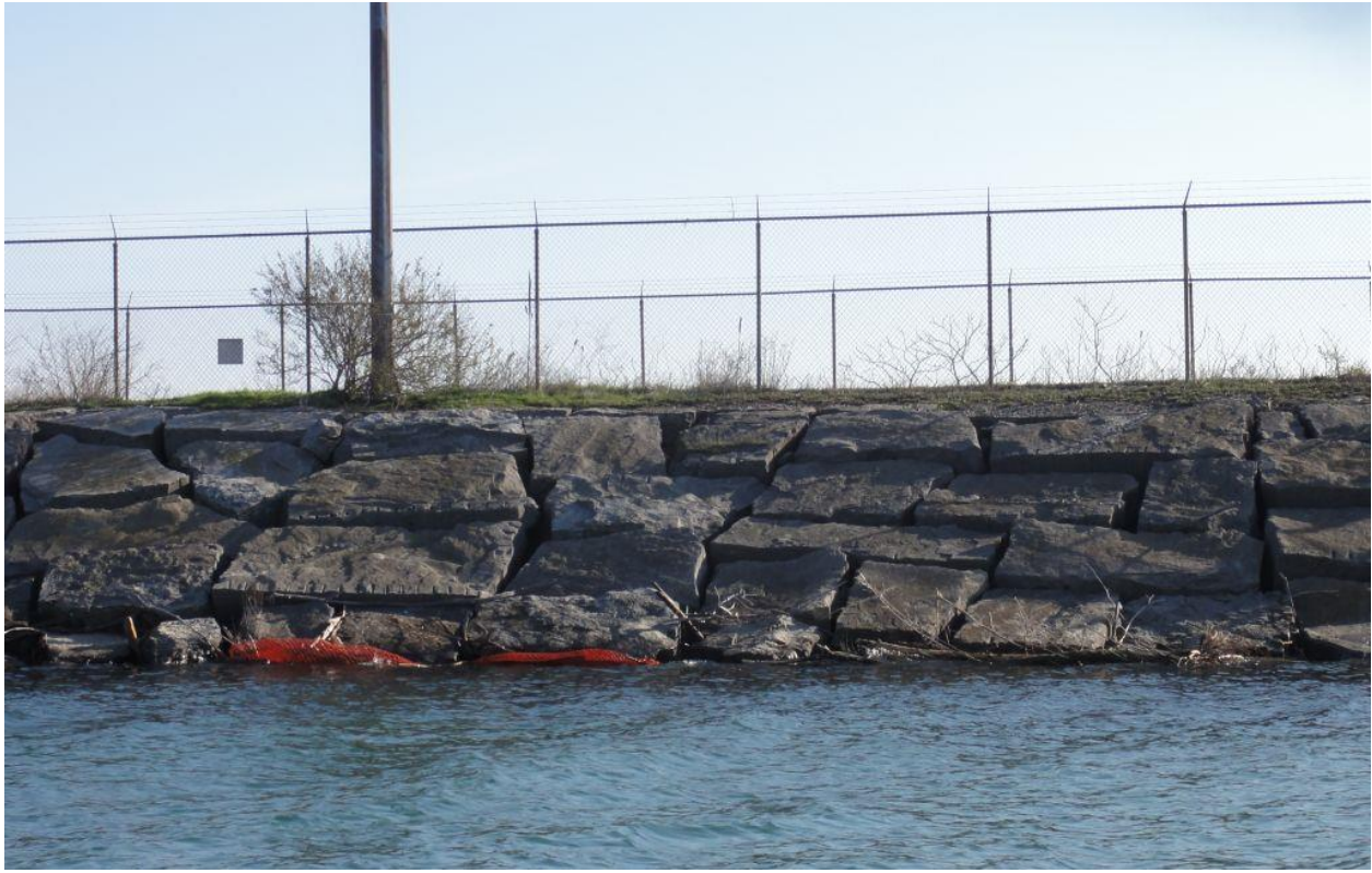
Figure 2.36: View from water of large, tightly placed armour stone on west side of Western Pier rubble mound mole
