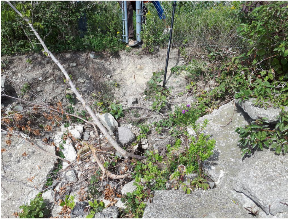
Figure 2.32: Localized wave uprush erosion at top of slope at westerly portion of Outer Shore
