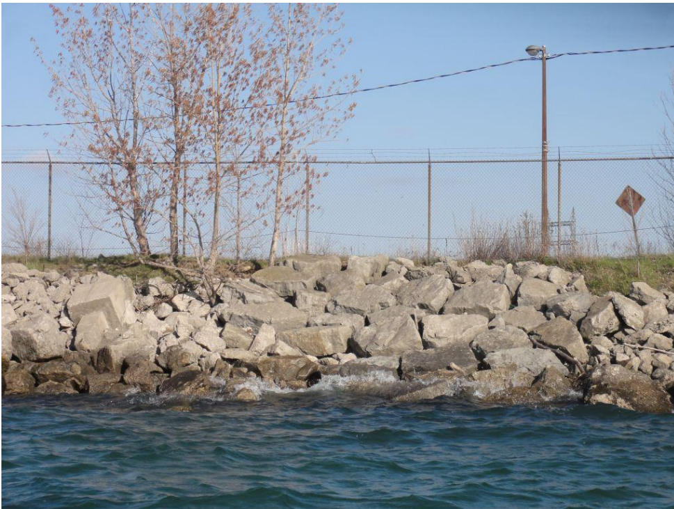
Figure 2.31: Example of additional armour stone on shoreline protection at westerly portion of Outer Shore
