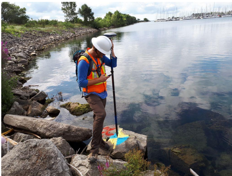
Figure 2.10: Baird survey of ground control points for UAV survey
