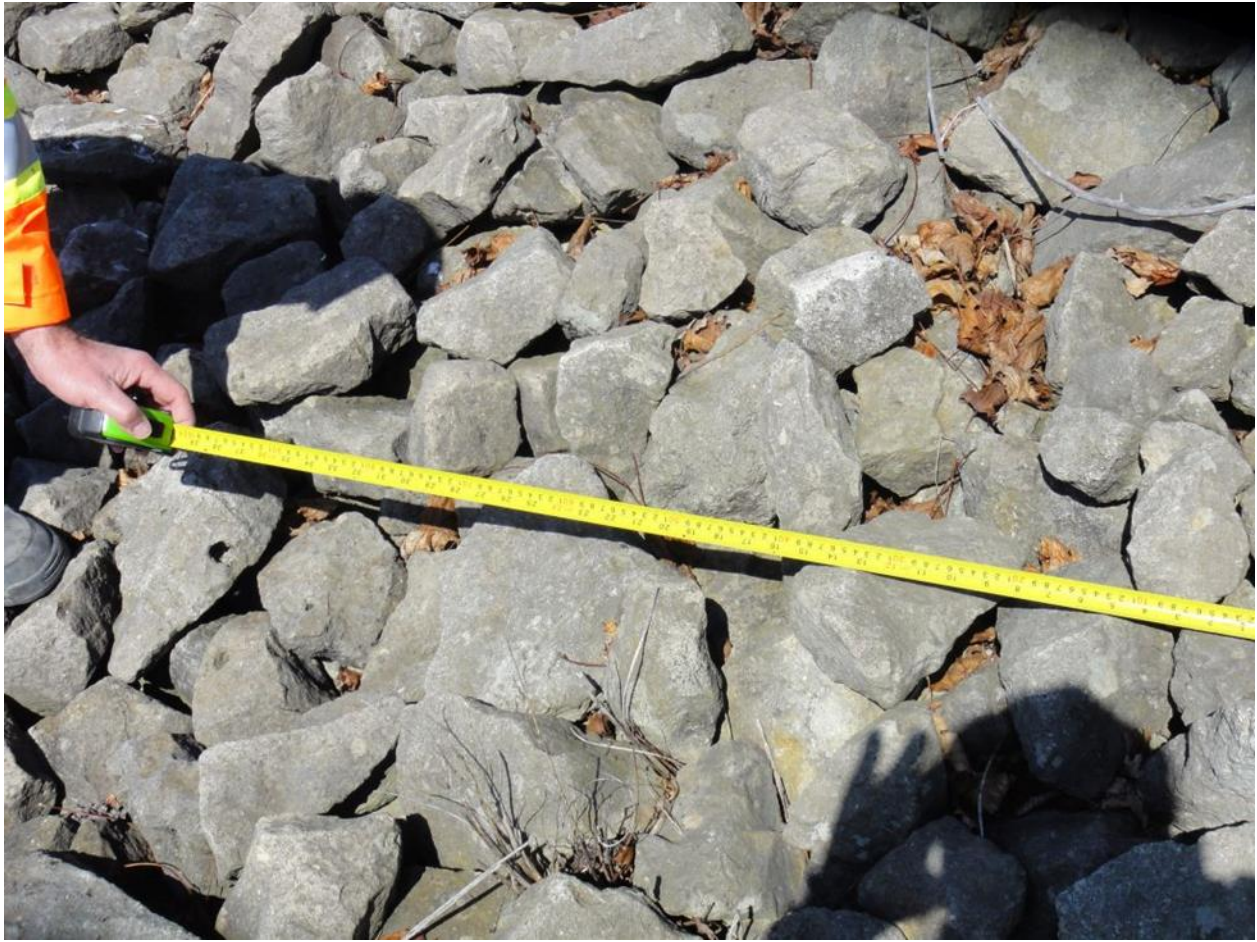
Figure 2.53: Example of riprap stone size at revetment along Intake Forebay/Channel North (between IFN660 and IFN735)
