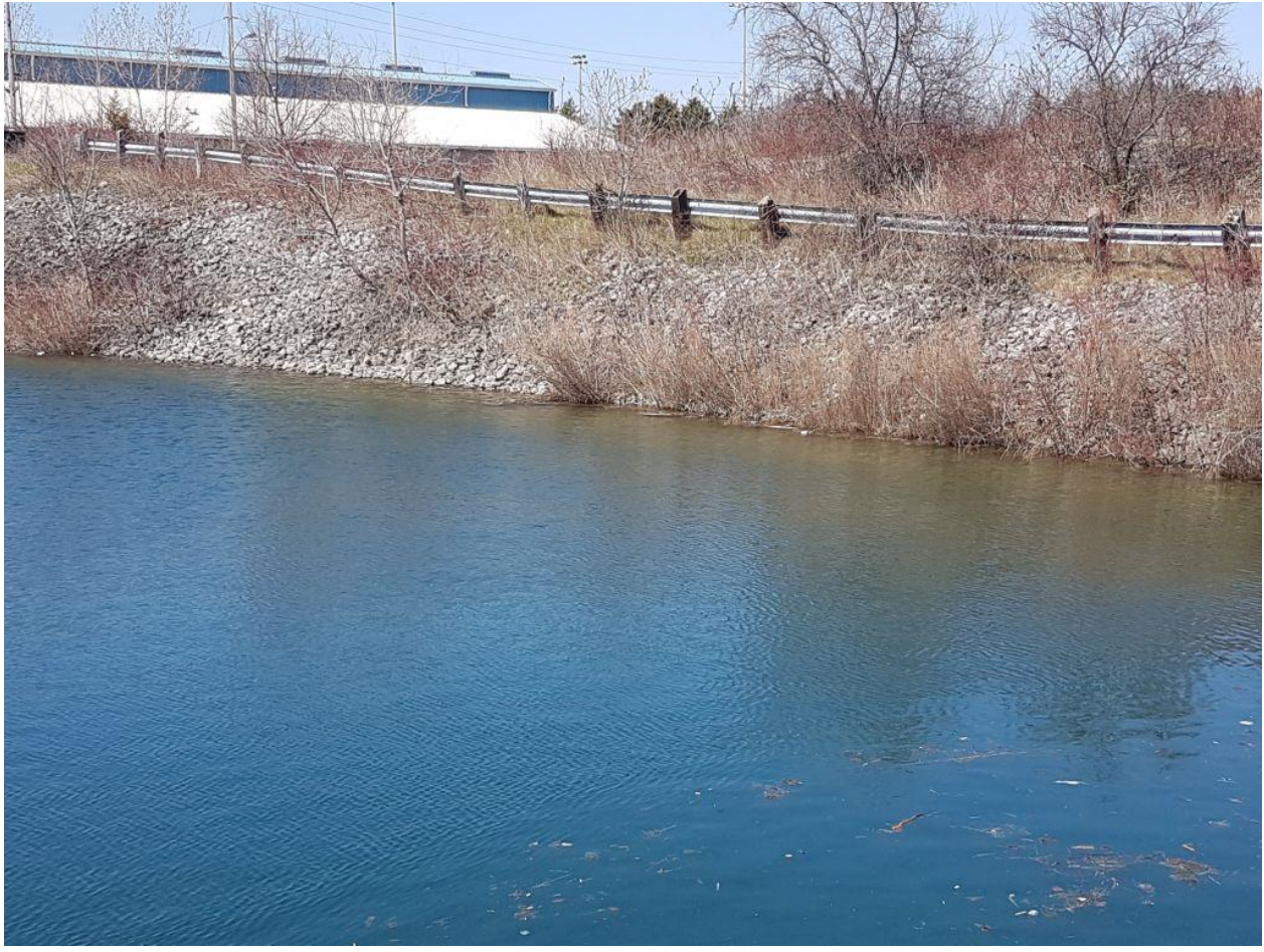
Figure 2.46: Discharge Channel West – vegetated riprap slope
