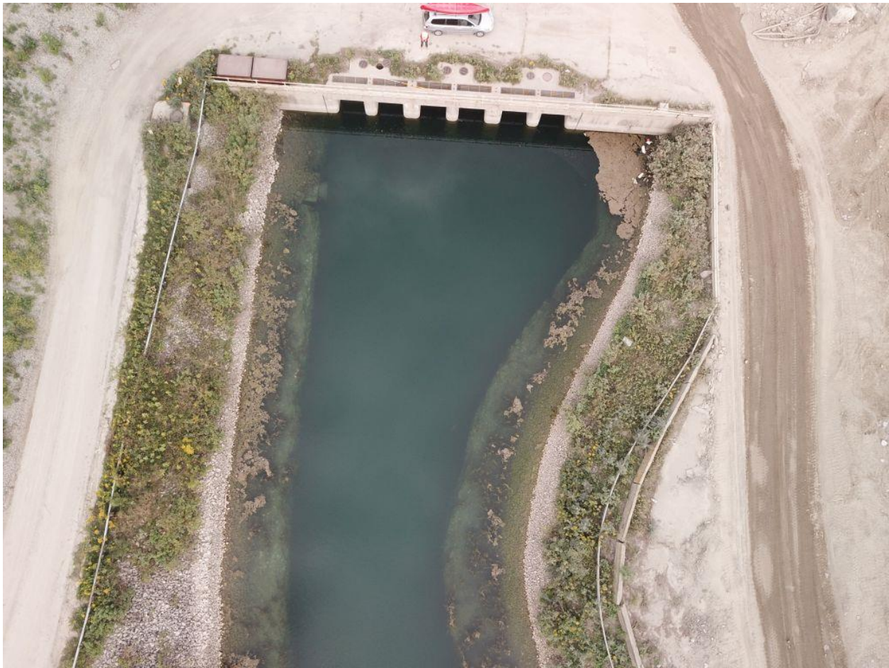
Figure 2.42: Headwall for discharge tunnels (Units 1 to 6) and channel excavated into bedrock
