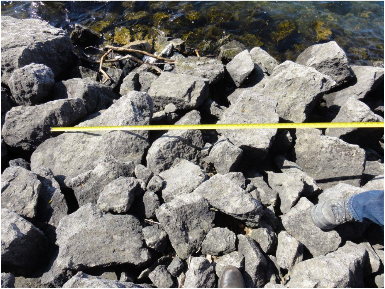
Figure 2.56: Larger riprap stone size along IFN shoreline nearer entrance
