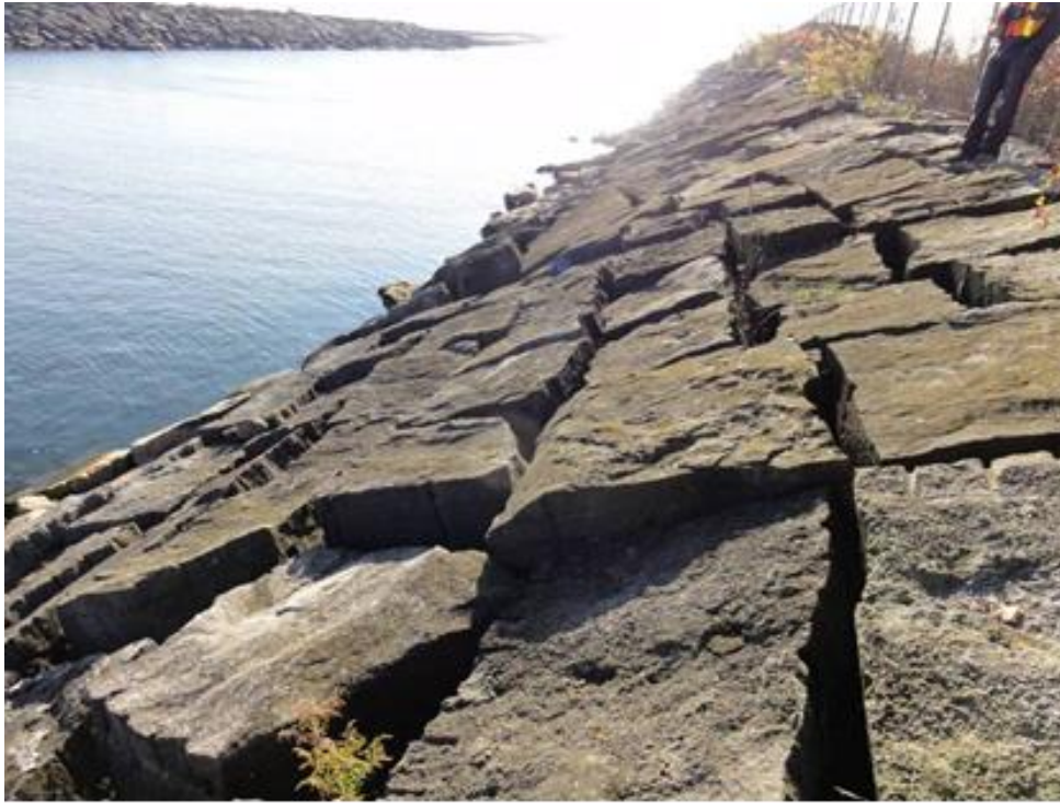
Figure 2.82: Typical section on east side of rubble mound mole portion of Western Pier
