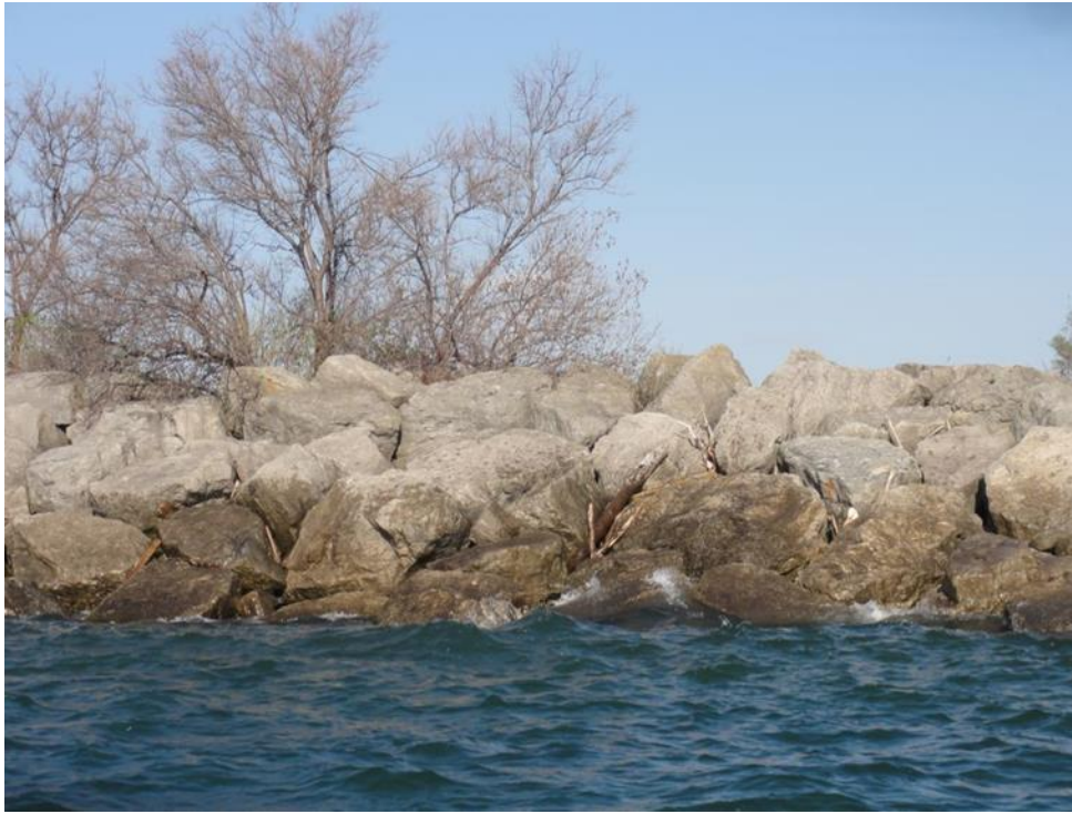
Figure 2.34: View from water of armour stone protection at Lakefront Promenade Park marina breakwater
