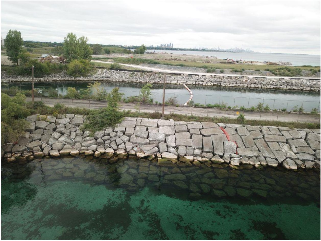
Figure 2.35: Tightly placed armour stone on west side of shore-end of Western Pier rubble mound mole
