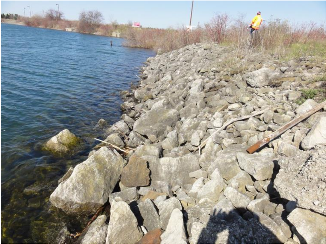
Figure 2.55: Intake Forebay/Channel North – larger riprap slope protection near easterly end, closer to entrance channel between piers
