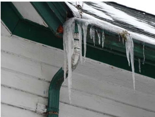
Rear Gable Temporary Repaired Downspout
