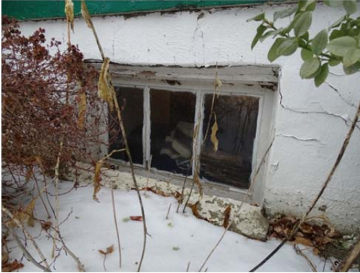
Exterior Foundation Showing Heavy Parging at Side
