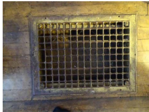
Return Air Register in Hardwood Floor at Entry
