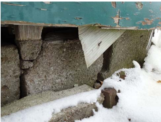
Failed Block Foundation Wall Under Porch
