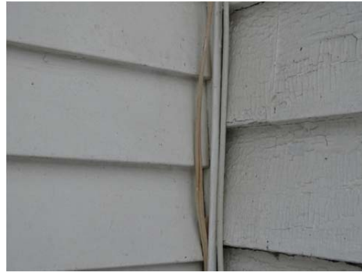
Wood Siding Meeting Smaller Metal Siding of the Tail.
