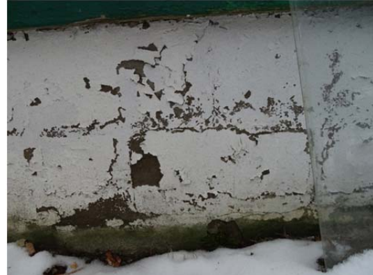
Foundation Wall at Front Showing Failed Light Parging
