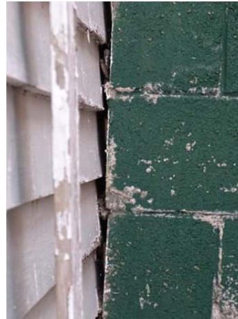
Gap Between Chimney and Siding
