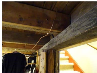
Sistering of Alternate Floor Joists
