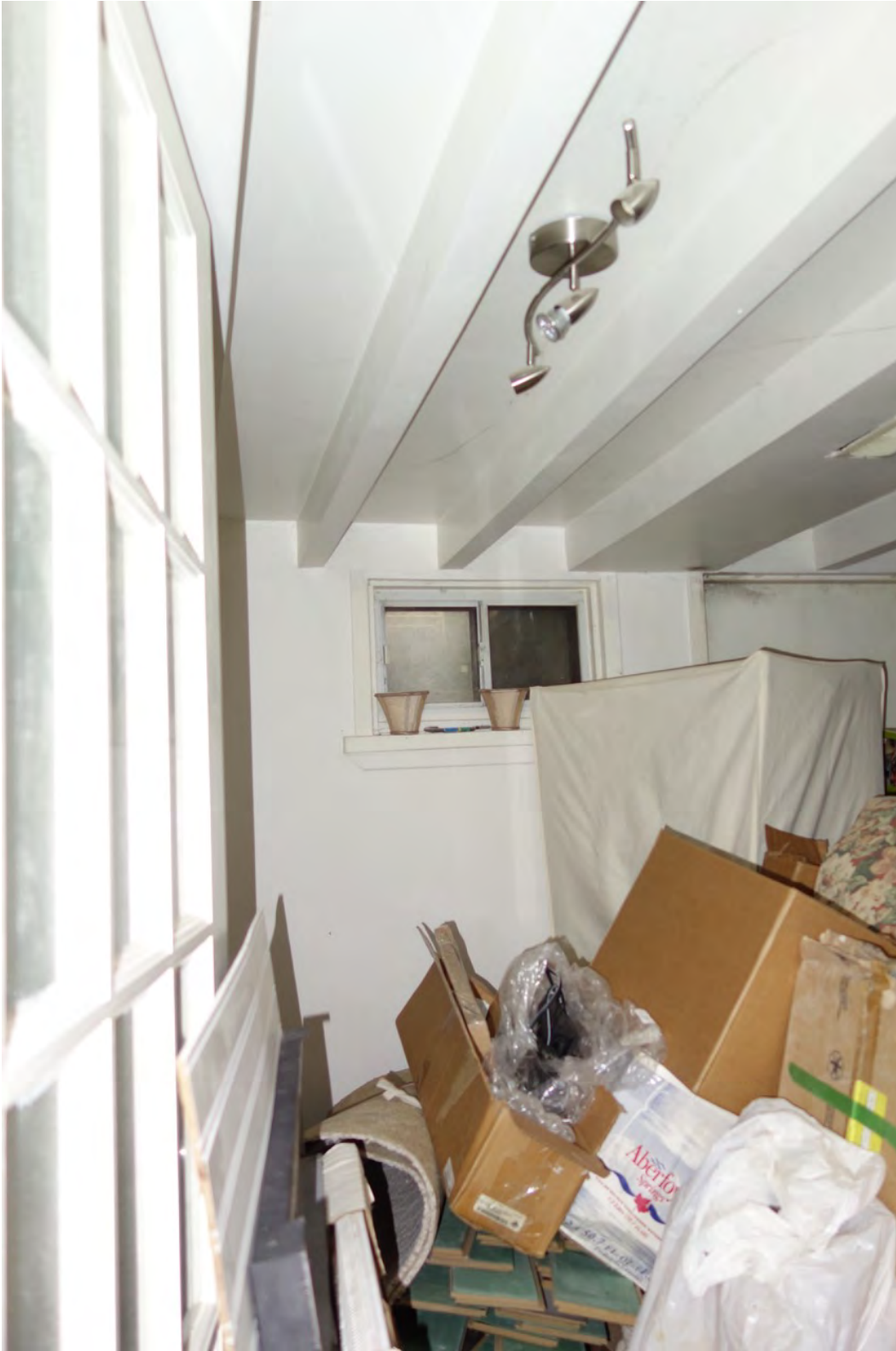
Figure 43: 24 Ann Street - INTERIOR – BASEMENT – storage room - exposed beams with modern spray stucco finish – modern window
