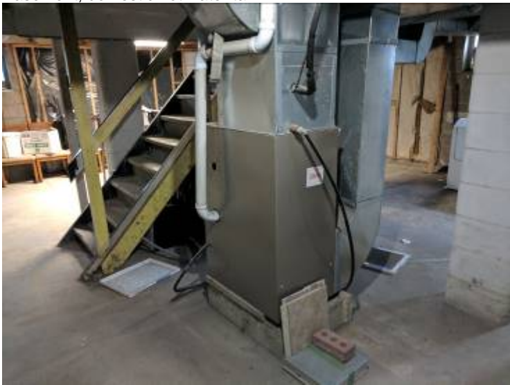
Gas-fired furnace in basement
