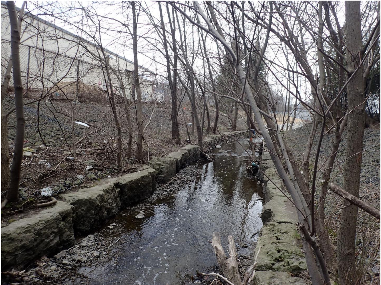
Photo G: Creek corridor mid-way between St. James Ave. and Lakeshore Rd. E. Photo taken facing south. Note that the creek bed and valley slopes consist of gabion baskets.
