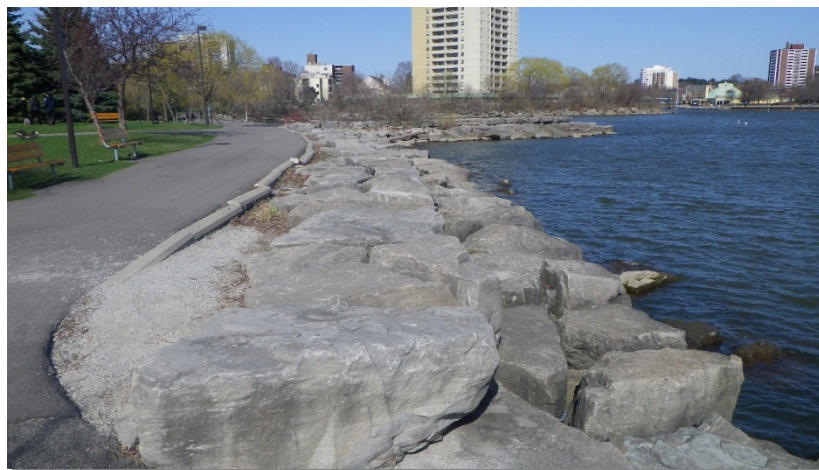
A34: Armour Stone Along J.C. Saddington Park, East Side
