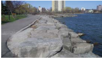
Stacked Armour Stone Wall J.C. Saddington Park
