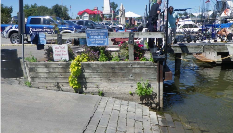
Photo A 22 - Launch Ramp, Timber and Steel Sheet Pile Walls in Marina Park
