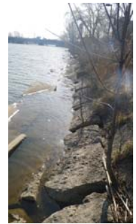
Concrete Slab Revetment Port Credit Memorial Park (West)
