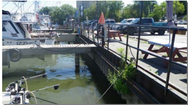
A20: Steel Sheet Pile Wall in Marina Park
