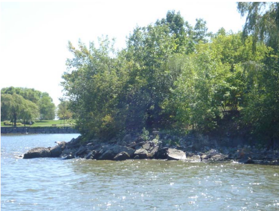
Photo A 28 – Armour Stone/Rubble Revetment along Rivergate Easement
