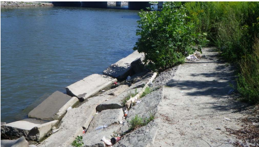
Photo A 9– Concrete Slab Shore Treatment along Memorial Park (West)
