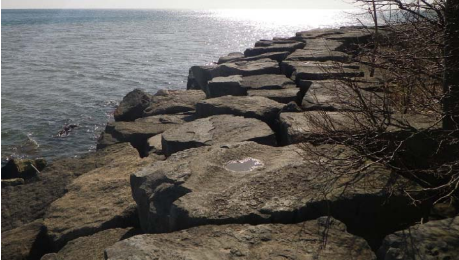
Photo A 35 – Armour Stone along J.C. Saddington Park, South East Side
