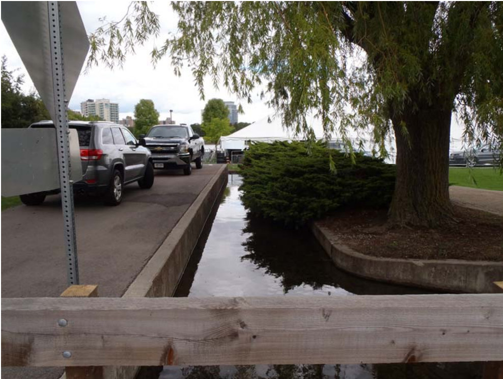
Photo 4 – Concrete outlet channel from pond flowing into naturalized outlet
