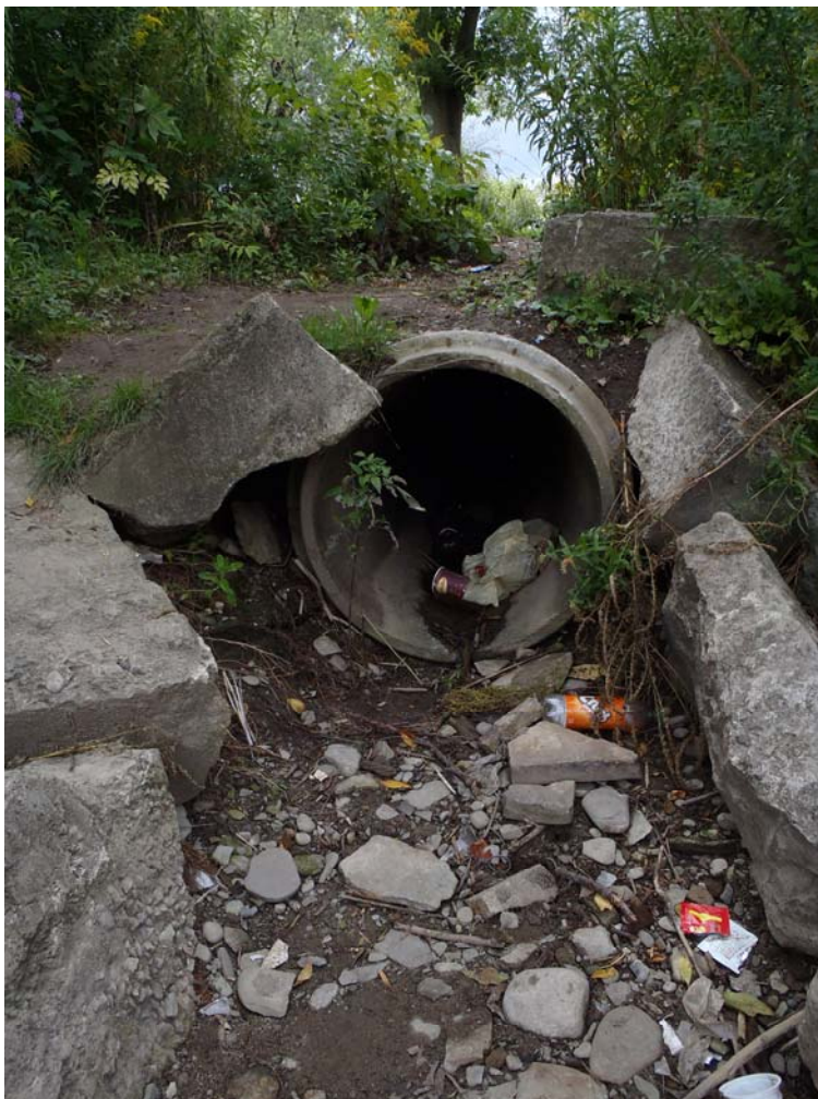
Photo 9 – Storm outfall (675mm) at Memorial Park West north of Lakeshore Road
