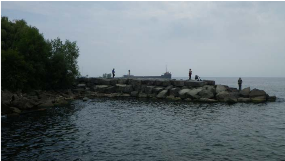
Photo A 36 – Armour Stone along J.C. Saddington Park, South East Headland
