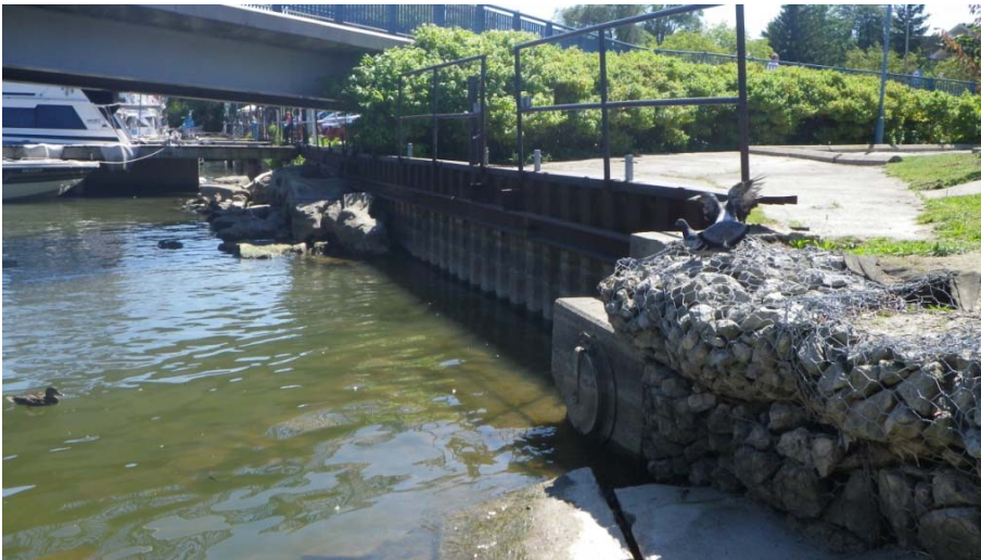
Photo A 17 – Gabion Basket and Steel Sheet Pile Walls South of Lakeshore Rd. Bridge
