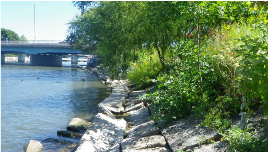
Photo A 8 – Concrete Slab Shore Treatment along Memorial Park (West)
