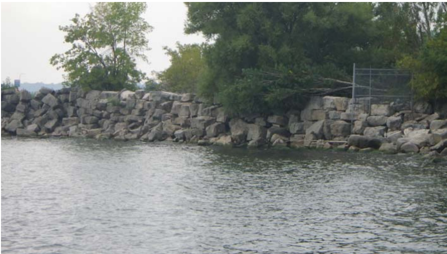
Photo A 41 - Armour Stone Pier West of J.C. Saddington Park
