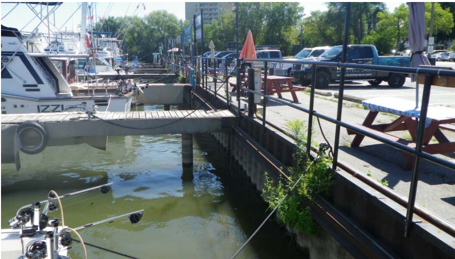
Photo A 20 – Steel Sheet Pile Wall in Marina Park
