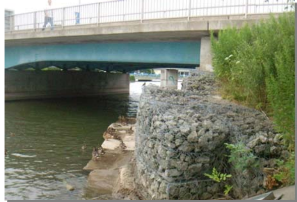
A14: Gabion Wall and Lakeshore Road Bridge
