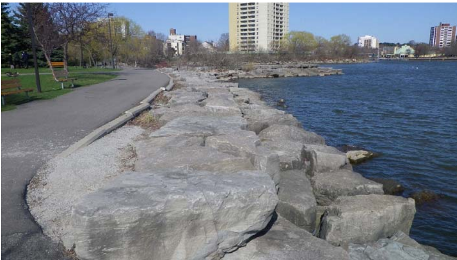
Photo A 34 – Armour Stone along J.C. Saddington Park, East Side
