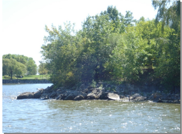
A28: Armour Stone/Rubble Revetment along Rivergate Easement
