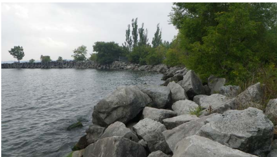
Photo A 39– Armour Stone/Rubble Revetment along J.C. Saddington Park, South Side
