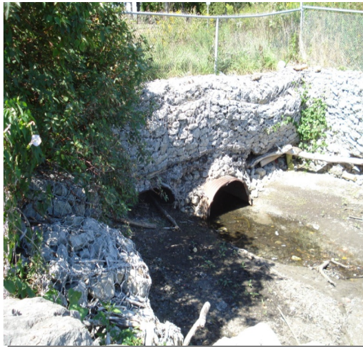
A40: Storm Sewer Outlets at West of J.C. Saddington Park
