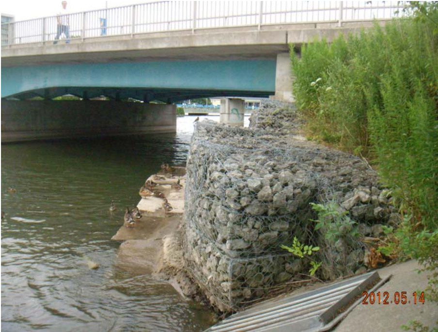
Photo A 14 - Storm Sewer Outlet, Gabion Wall and Lakeshore Road Bridge
