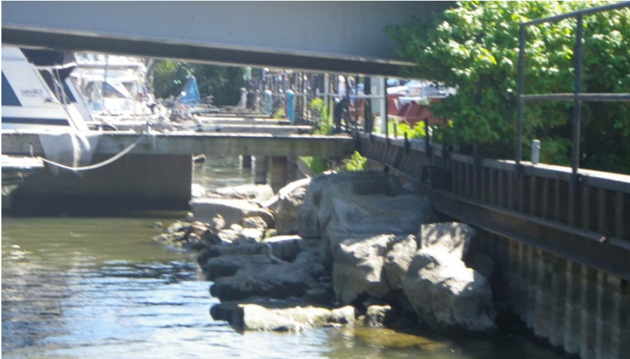
Photo A 19 – Armour Stone Revetment & Steel Sheet Pile Wall in Marina Park
