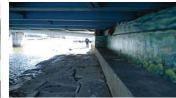
Lakeshore Road Bridge Abutment with Armour Stone Revetment
