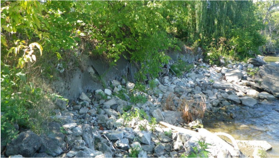
Photo A 29 – Failed Revetment along Rivergate Easement
