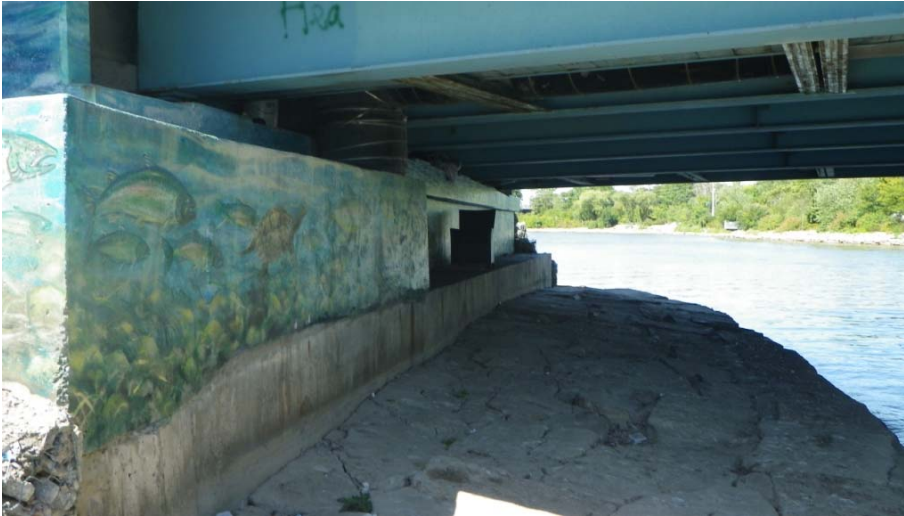
Photo A 16 – Shore Treatment and Abutment, Lakeshore Road Bridge
