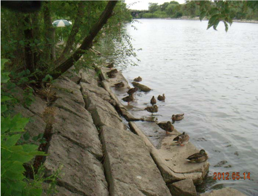
Photo A 10– Concrete Slab Shore Treatment along Memorial Park (West)
