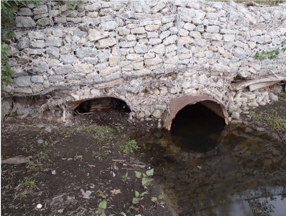
Photo 1 - Close up view of outlet structure at the extension of Mississauga Road
