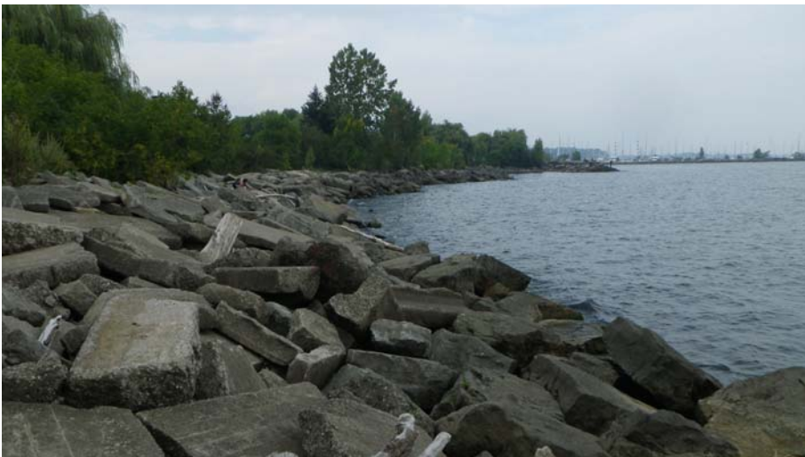
Photo A 37 – Rubble Revetment along J.C. Saddington Park, South Side
