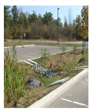
Figure 6-16: The drainage for the parking area at Riverwood Park has been designed to mimic natural ecological functions such as water infiltration and purification. The runoff from this bio-swale outlets to a small wetland feature on the park site.
