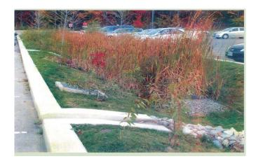
Figure 9-34: Bio-retention features, such as **stormwater best management practices**, are encouraged to be incorporated in site development.
