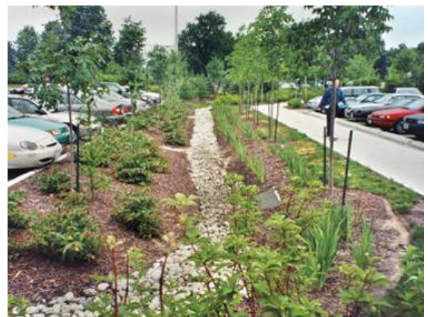
Figure 24: Boulevards in parking areas should incorporate soft landscape materials and shade trees with design elements and systems that mitigate storm water run-off.
