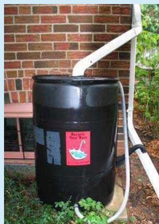
Figure D3 — Typical rain water barrel
