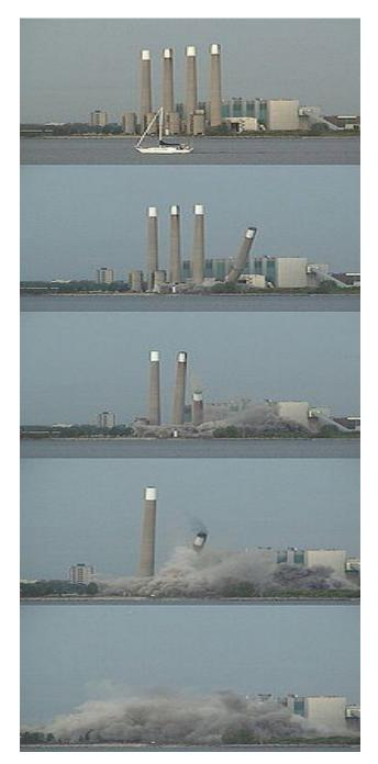
Figure 19-6: The Lakeview Generating Station, also known as the Four Sisters, ceased operations in April 2005 after 43 years and was demolished in June 2006. The former coal burning station had been in operation since the early 1960's.
