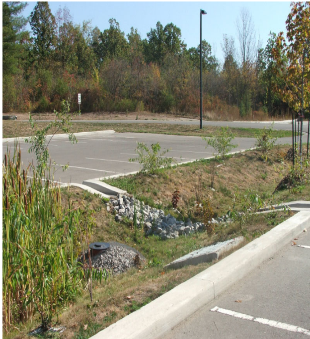
Figure 6-17: The drainage for the parking area at Riverwood Park has been designed to mimic natural ecological functions such as water infiltration and purification. The runoff from this bio-swale outlets to a small wetland feature on the park site.
