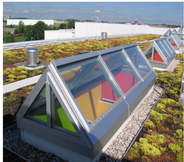
Figure 9-38: Green roofs are an effective stormwater best management practice and contribute to the reduction of the urban heat island effect.
