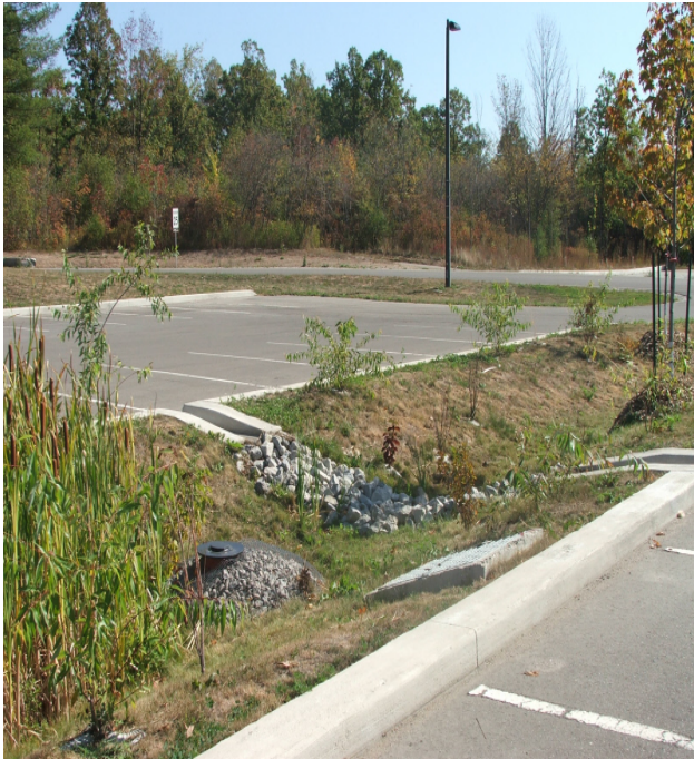
Figure 6-16: The drainage for the parking area at Riverwood has been designed to mimic natural ecological functions such as water infiltration and purification. The runoff from this bio-swale outlets to a small wetland feature on the park site.
