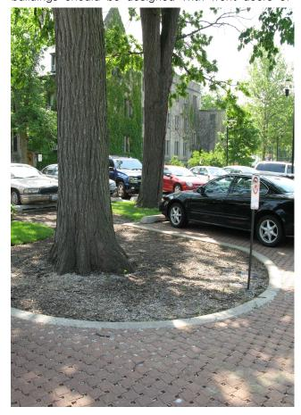
Figure 9-33: Permeable paving is used to enhance tree preservation efforts and to promote stormwater infiltration at Dominican University, in River Forest, Illinois.
