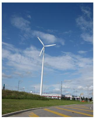
Figure 10-11: A 31 m wind turbine unveiled at the Lisgar GO Station in April 2009, generates as much as 80 per cent of the station's power. The site, located at Tenth Line and Argentia Road, was chosen for the wind turbine because of heavy prevailing winds from the west and its open fields.
