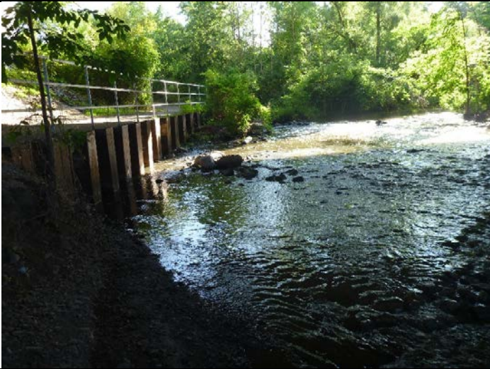
Photo 37: View of the pathway and sheet pile under the Mavis Road bridge
