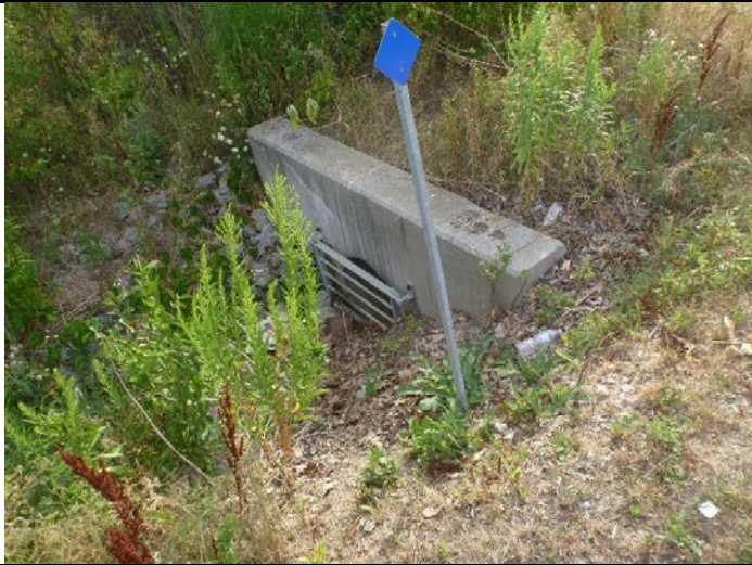
Photo 13: Storm Inlet located at the east side of Mavis Road where the Hwy 407 S-E Ramp start.
