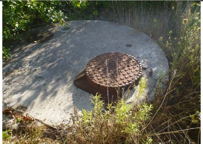
Photo 42: SWM facility no. 4 – Storm outlet control manhole
