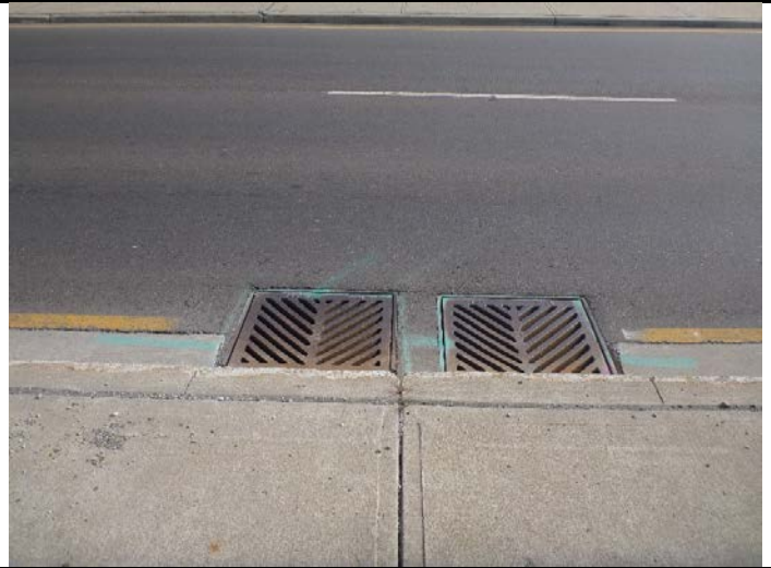
Photo 14: Catch basin along the south Bound of Mavis Road where Mavis Road Storm Sewer System start
