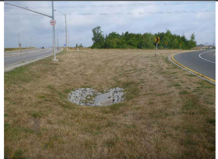
Photo 10: Looking north, Ditch Inlet located between Mavis Road and Hwy 407 S-E Ramp
