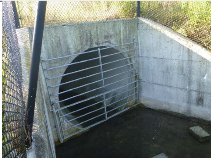
Photo 45: SWM facility no. 4 – Bypass outlet
