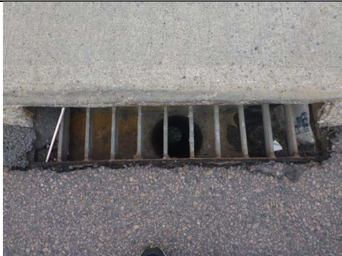
Photo 51: Inlet along Mavis Road bridge that drain into Fletcher's Creek directly
