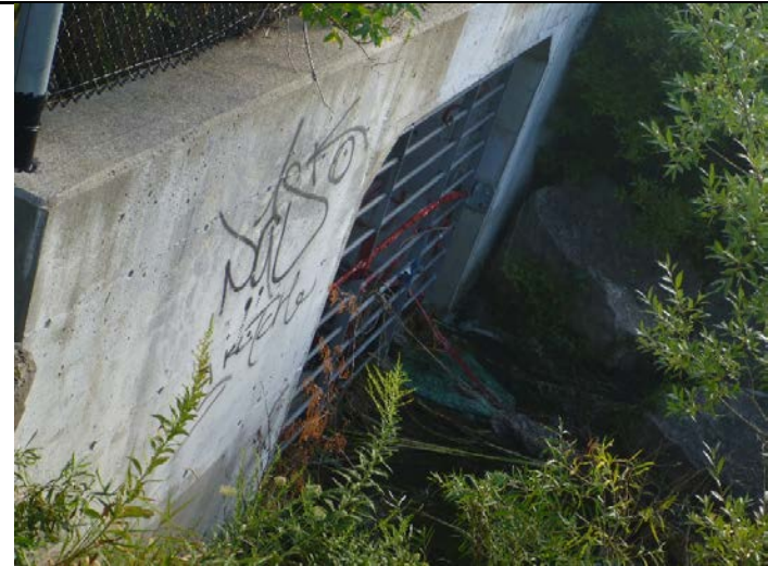
Photo 28: SWM facility no. 5 – Outlet structure, headwall in the downstream face.
