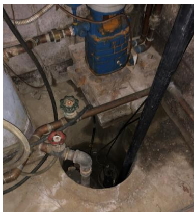
Picture 8: View of the basement sump located in 1240 Britannia Road.
