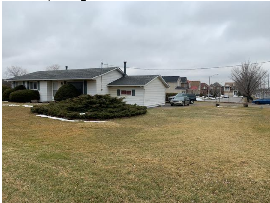
Picture 3: View of the east side of the house at 1310 Britannia Road, facing southwest.
