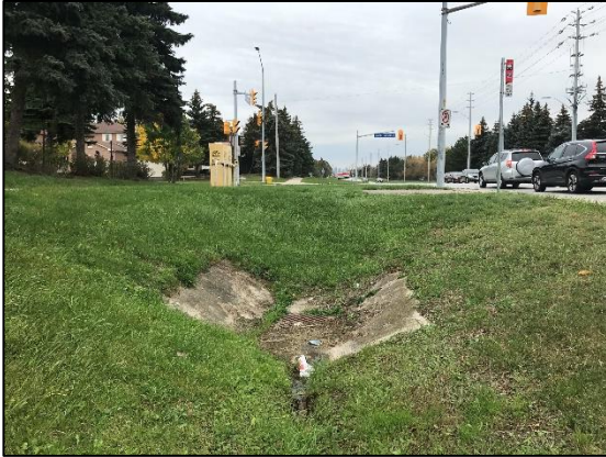
Image 13: Field Conditions, Showing Ditching and Ditch Inlet Catch Basin, Facing Southwest
