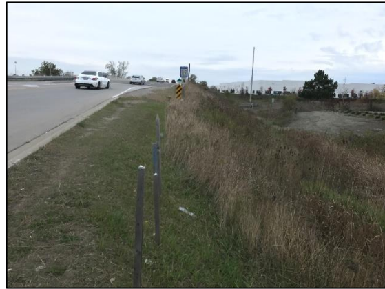
Image 22: Field Conditions, Showing Study Corridor, Facing Northeast
