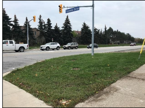
Image 14: Field Conditions, Showing Study Corridor at Colonial Drive, Facing West
