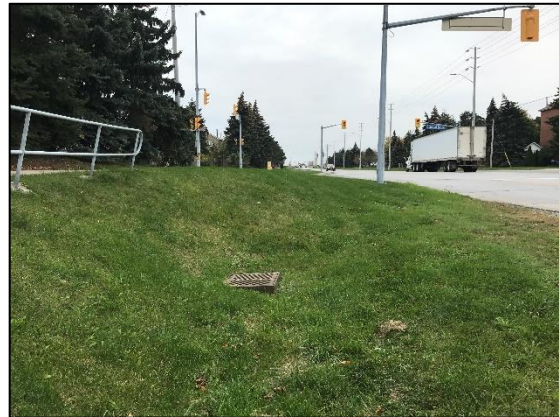
Image 12: Field Conditions, Showing Ditching and Ditch Inlet Catch Basin, Facing Northeast
