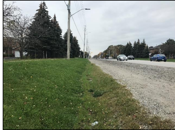
Image 8: Field Conditions, Showing Study Corridor, Facing Southwest
