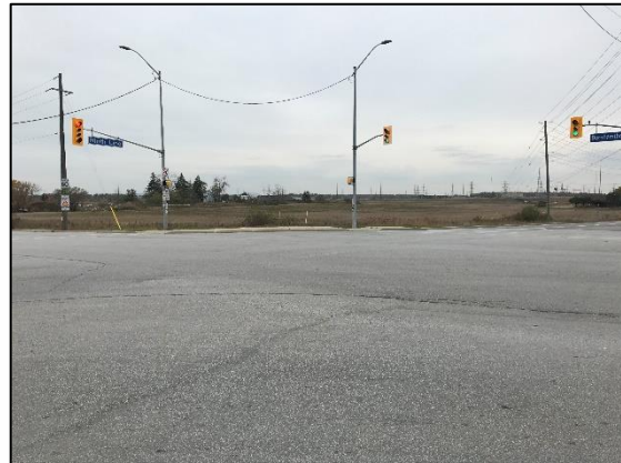
Image 24: Field Conditions, Intersection of Burnhamthorpe Road West and Ninth Line, Facing North
