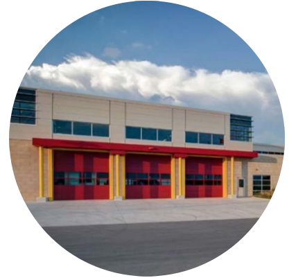
Garry W. Morden Fire Training Centre
