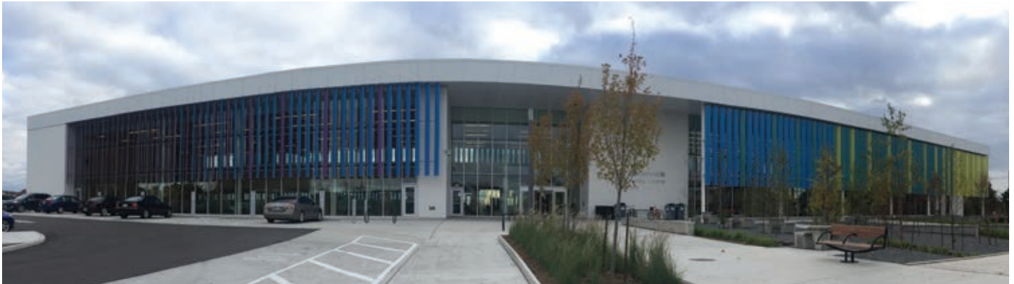
Meadowvale Community Centre and Library, front entrance.
