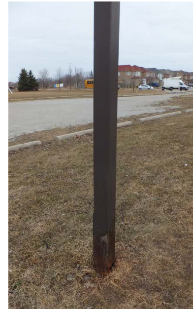
Pathway lighting pole replacement
