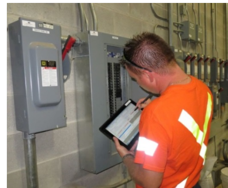
Facilities Maintenance staff utilizing HAT technology
