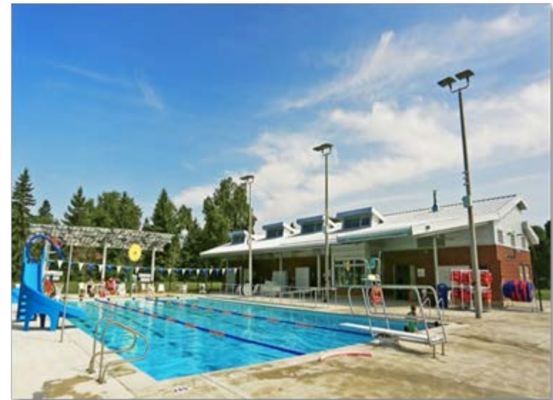
Don McLean Westacres Outdoor Pool (Completed in June 2014)
