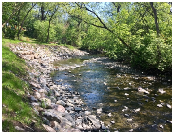
Watercourse bank stabilization at failed storm outfall
