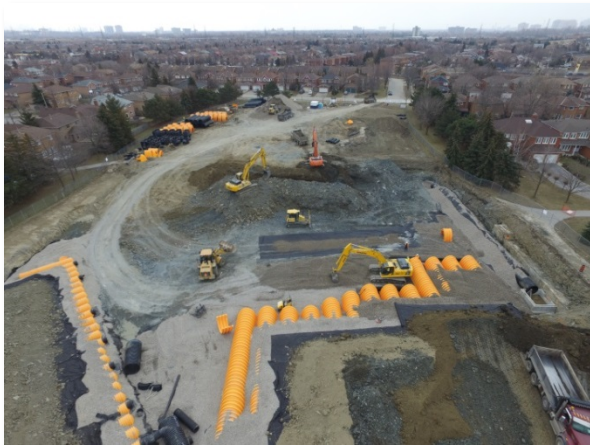
Installation of storage chambers at Eastgate Park
