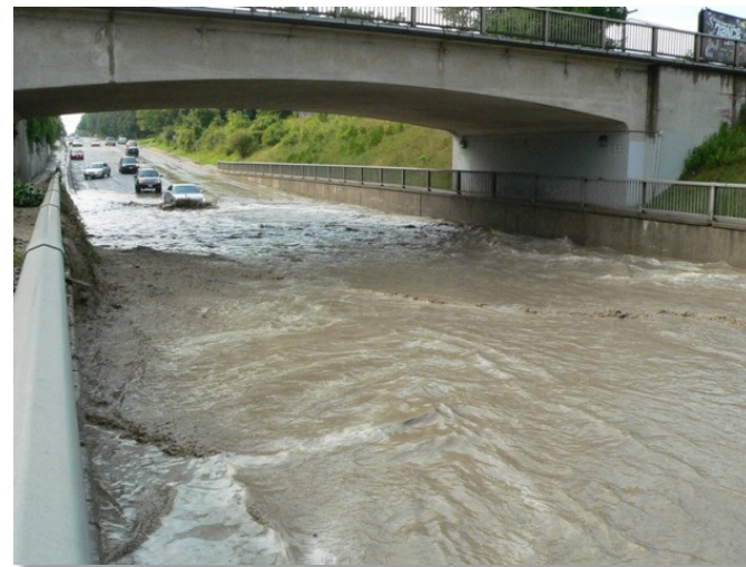
Flooding of rail underpass during an extreme storm event (source: Credit Valley Conservation)
