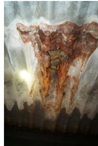
Corroded metal storm sewers require replacement
