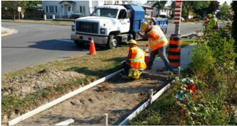
Sidewalk Repairs on Forestwood Drive
