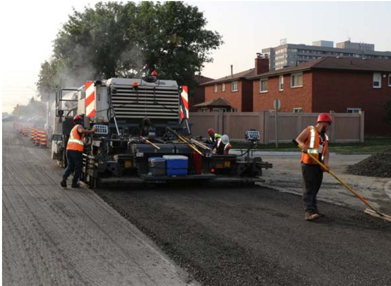
Asphalt Recycling on Central Parkway
