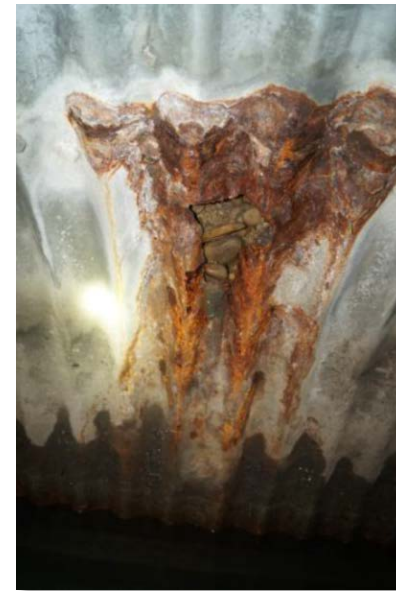
Corroded metal storm sewers require replacement
