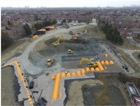
Installation of storage chambers at Eastgate Park
