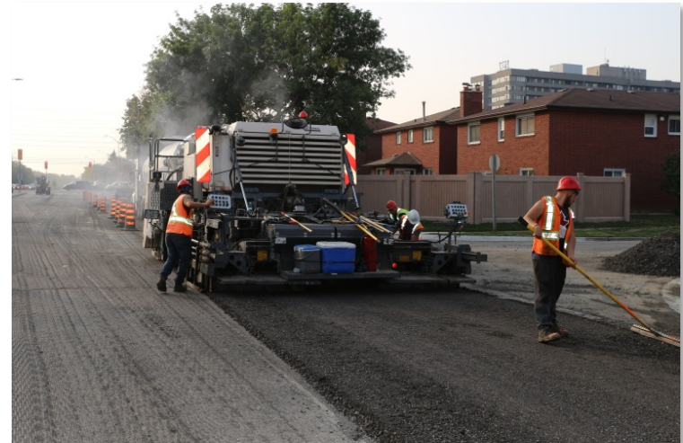
Asphalt Recycling on Central Parkway
