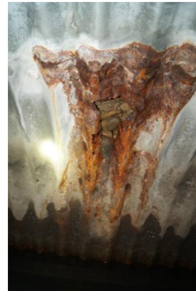
Corroded metal storm sewers require replacement
