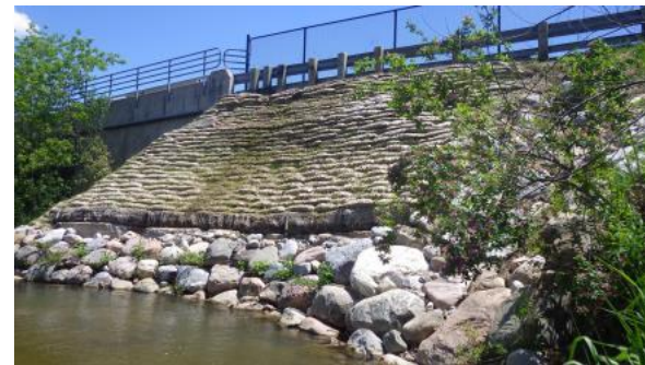
Watercourse slope stabilization at failed road embankment
