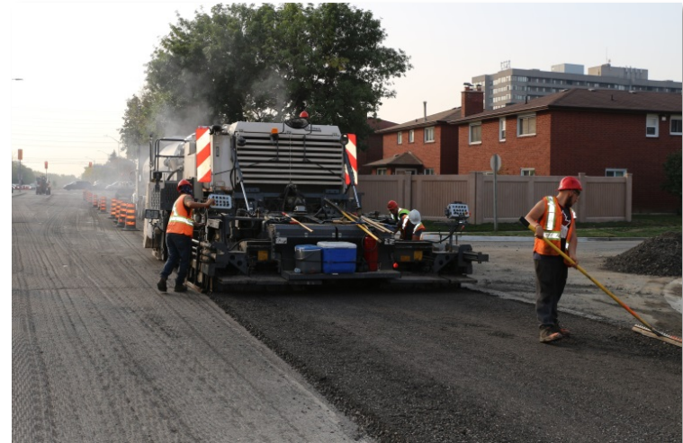
Asphalt Recycling on Central Parkway
