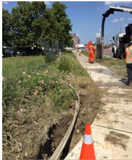
Installing conduits under road to bring the Internet and City IT services to Go Transit/TTC/MiWay's Renforth Gateway Terminal
