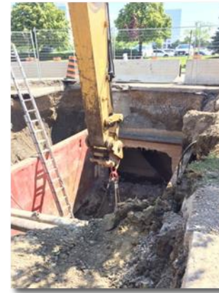
Installation of new storm pipe infrastructure
