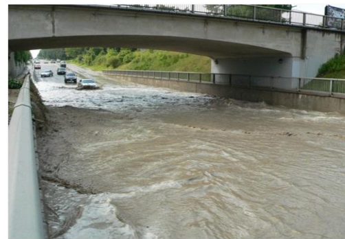
Flooding of rail underpass during an extreme storm event (source: Credit Valley Conservation)
