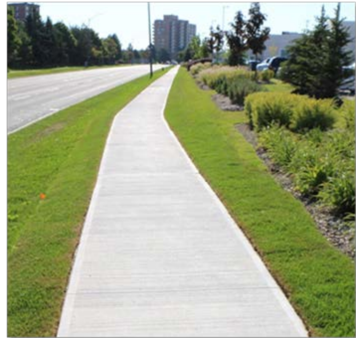
Newly Constructed Sidewalk on Ridgeway Drive
