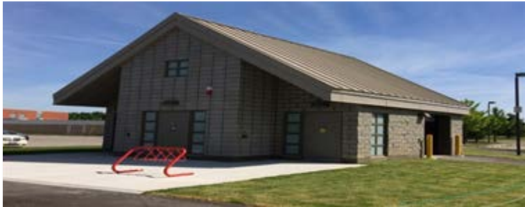
Community Park Washroom at Lisgar Fields Park
