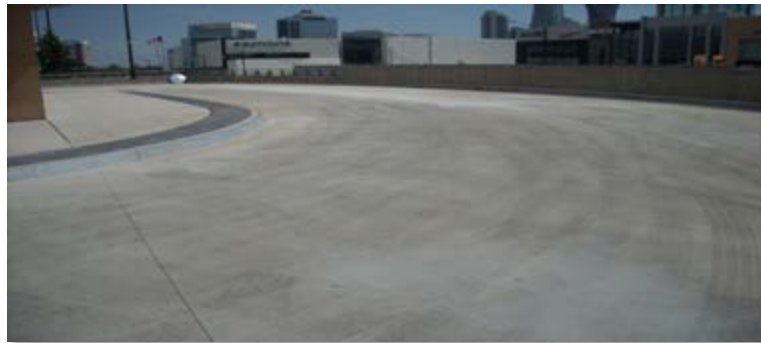
City Centre Transit Platform
