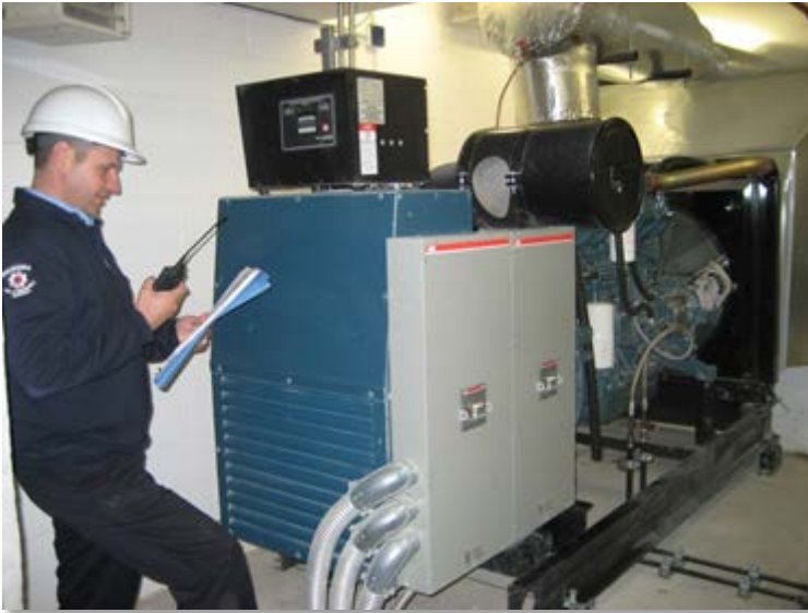
Inspecting Building Systems
