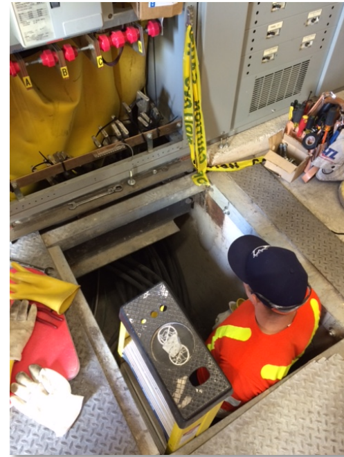
Facility Maintenance Staff performing emergency repair work
