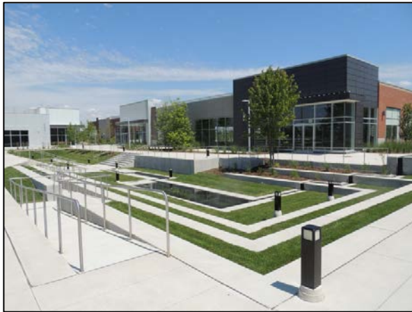
HOOPP Realty Inc. - Multi-Tenant Commercial Plaza (Spectrum Way and Eglinton Avenue East)
