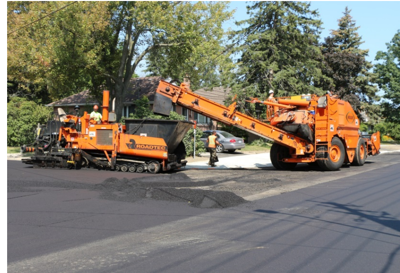
Atwater Avenue is one of many roads rehabilitated in 2015
