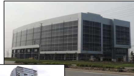
HOOPP Realty Inc. - Multi-Tenant Office Building (Prologis Boulevard and Hurontario Street)
