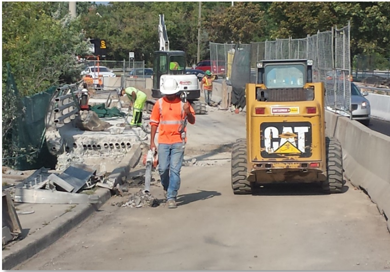
Bridge reconstruction on Burnhamthorpe Road East over Sawmill Creek
