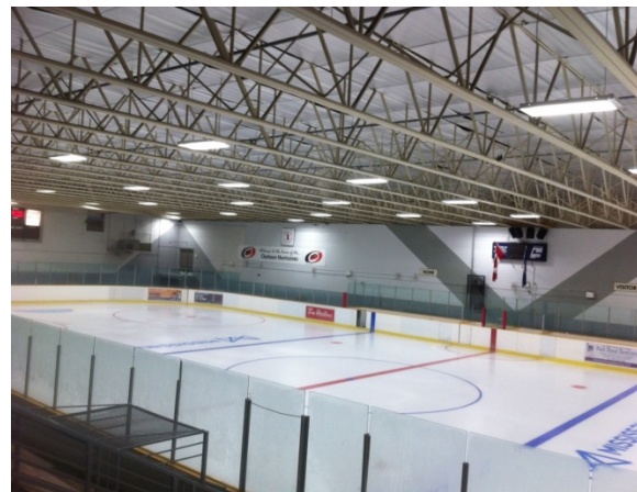
Clarkson Arena LED Light Retrofit Completed by F&PM.
