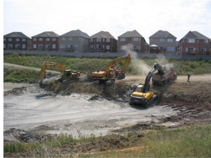
Stormwater Management Facility #5803 located southwest of Winston Churchill Boulevard and Artesian Drive is dredged of sediment
