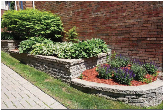
Figure 2.6: Landscape retaining walls should not be higher than 0.6 m
