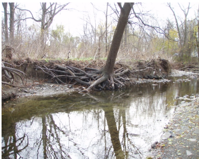
Figure 6-17: Erosion can result in serious danger to property, people, water resources, vegetation and infrastructure. Adherence to development standards and policies reduces these dangers and protects life and property.
