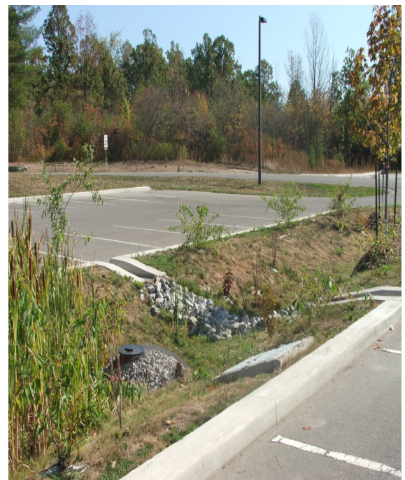
Figure 6-16: The drainage for the parking area at Riverwood Park has been designed to mimic natural ecological functions such as water infiltration and purification. The runoff from this bio-swale outlets to a small wetland feature on the park site.
