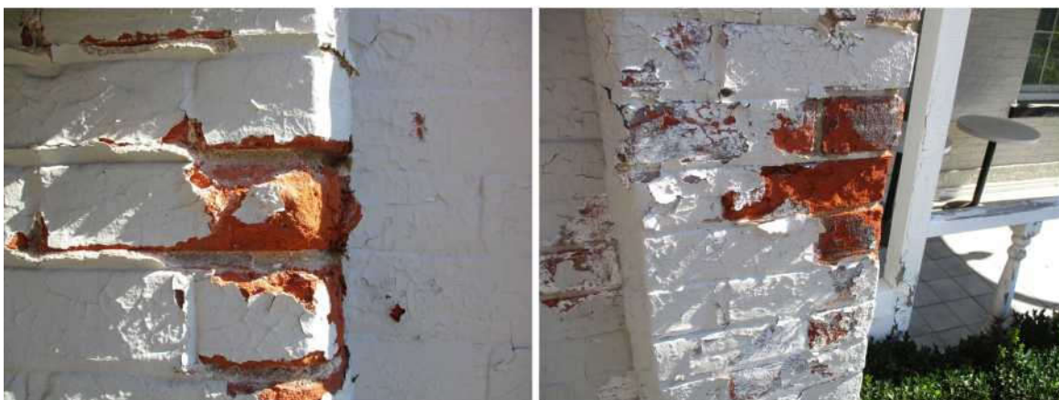
Figure 6a, 6b: Damage to masonry at south side of entry canopy
