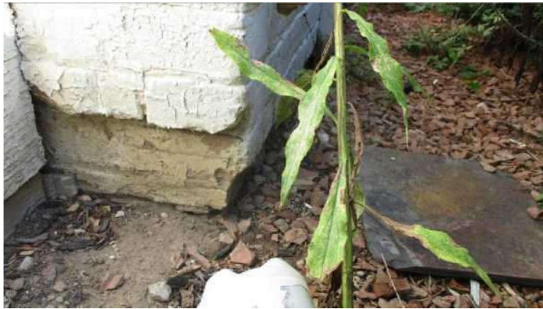
Figure 4: Deteriorated coatings near grade
