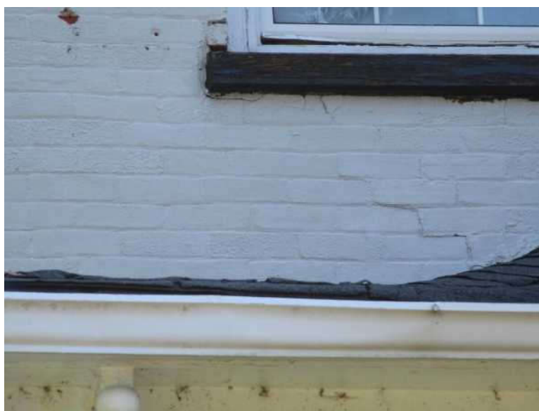
Figure 7: Step cracking below second storey window
