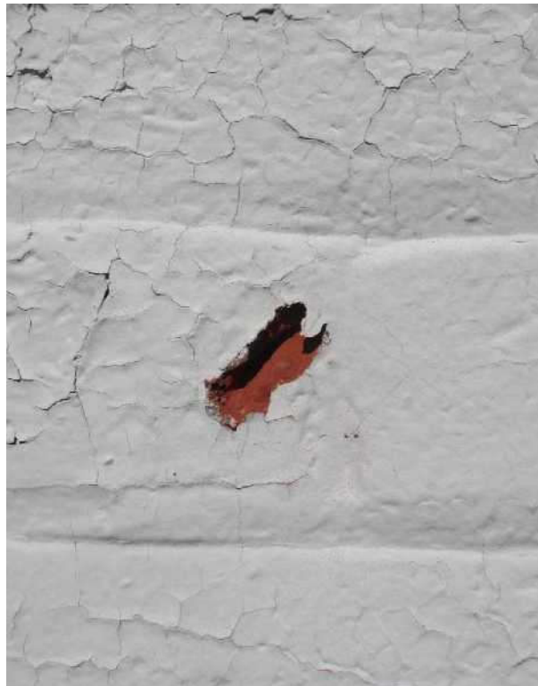
Figure 3: Soft brick exposed below coatings
