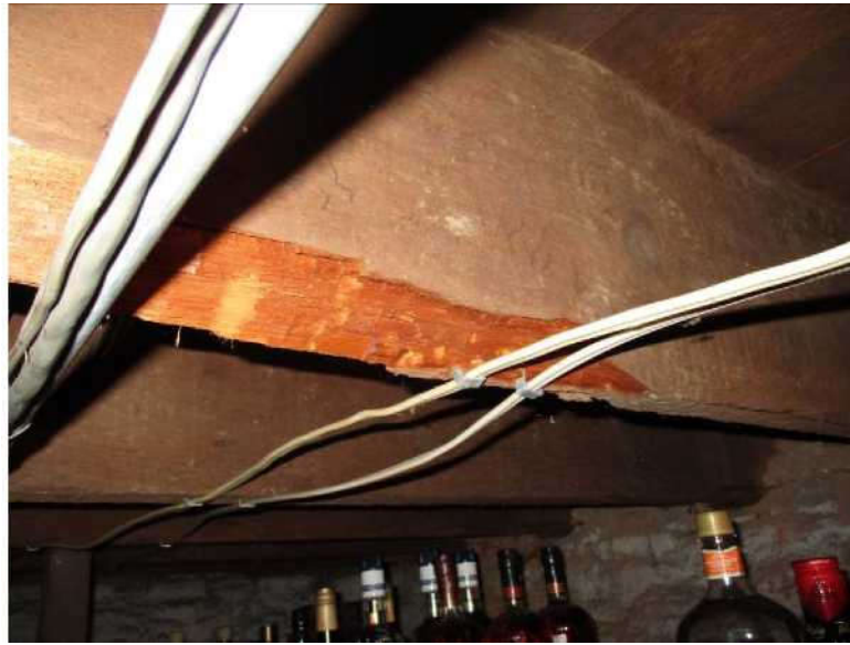
Figure 1: Deteriorated floor framing
