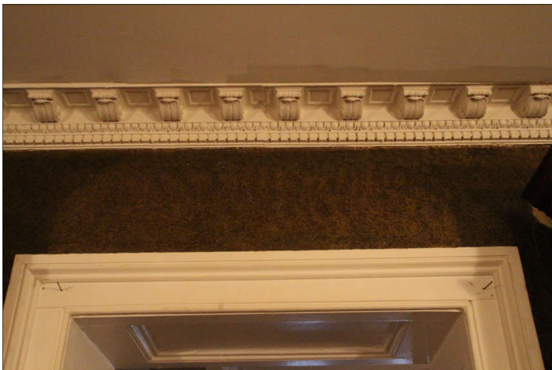
Figure 50 plaster ceiling moulding in current bar
