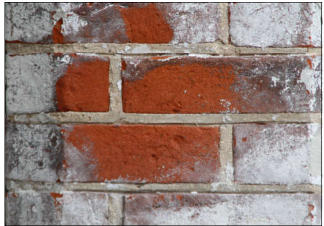
Figure 29 original red-orange brick under white paint
