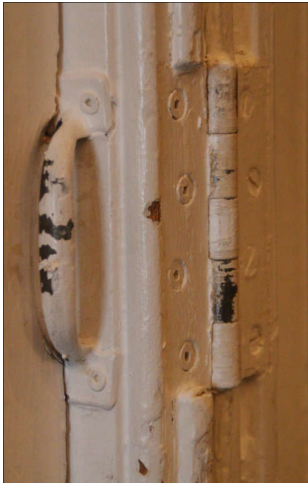
Figure 48 pocket door hinge & handle
