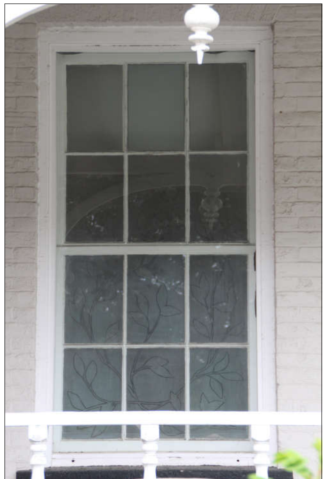
Figure 37 typical 6/6 sash window
