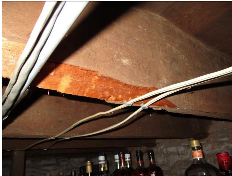
Figure 1: Deteriorated floor framing
