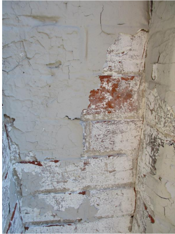
Figure 2: Exterior coatings
