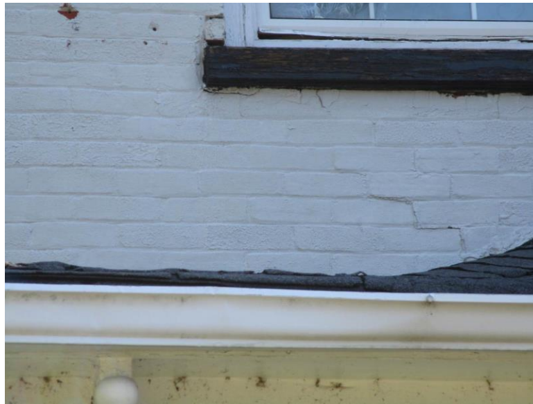
Figure 7: Step cracking below second storey window
