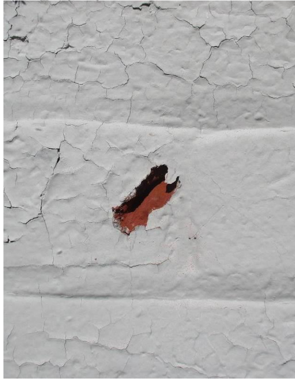
Figure 3: Soft brick exposed below coatings
