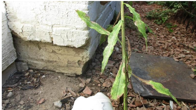
Figure 4: Deteriorated coatings near grade
