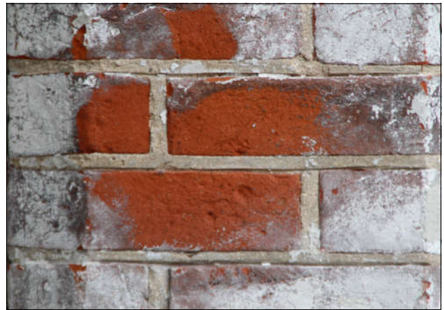
Figure 28 original red-orange brick under white paint
