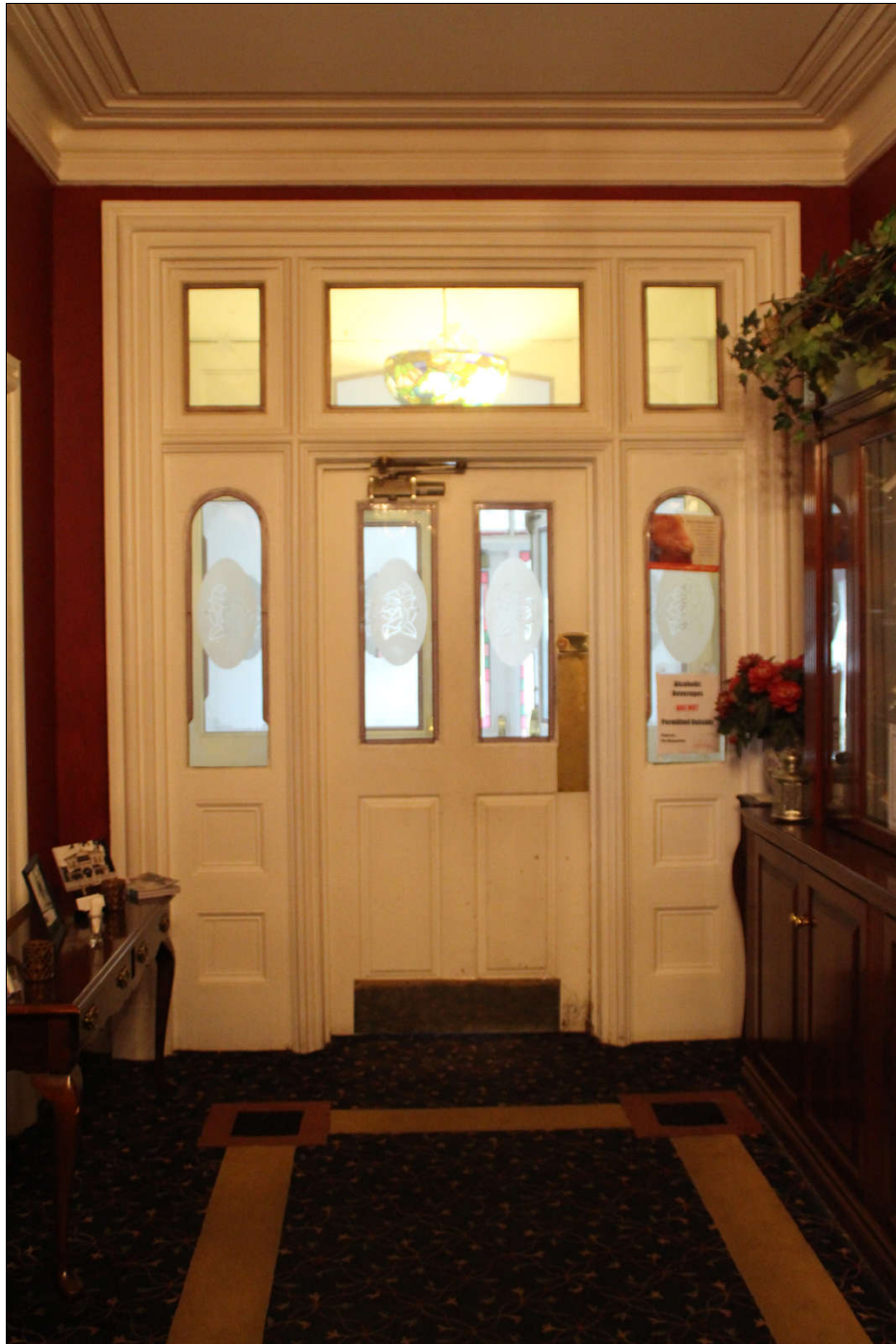
Figure 39 inside front door, transom & sidelights (replacement glass), ceiling moulding
