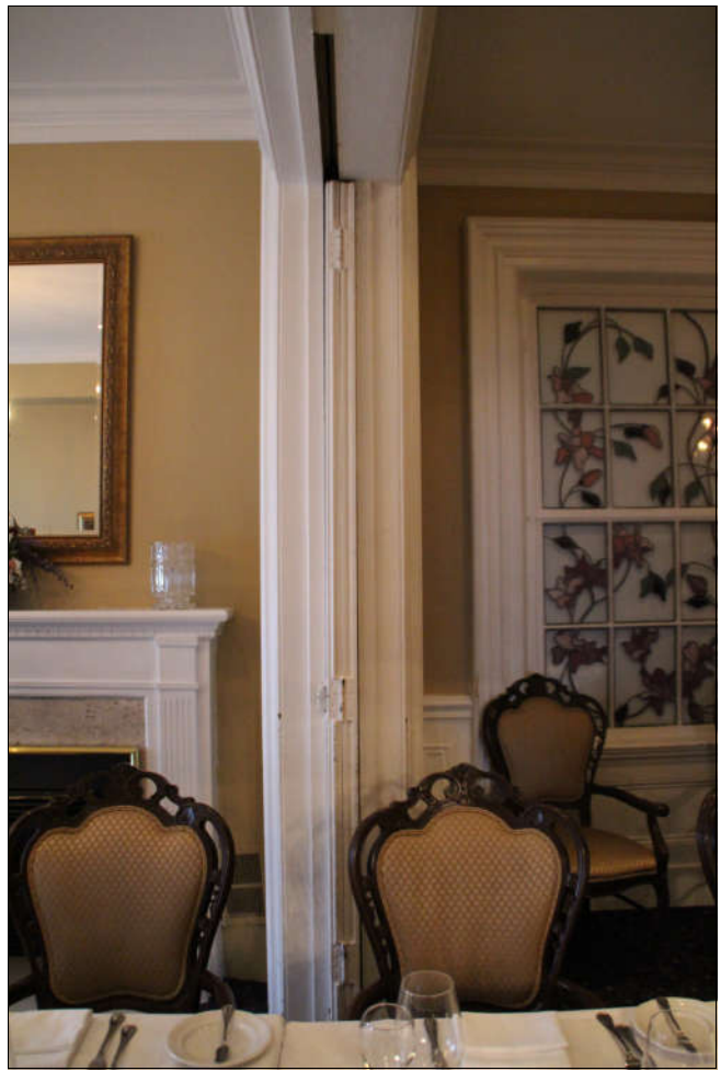
Figure 44 folding pocket doors between north parlours
