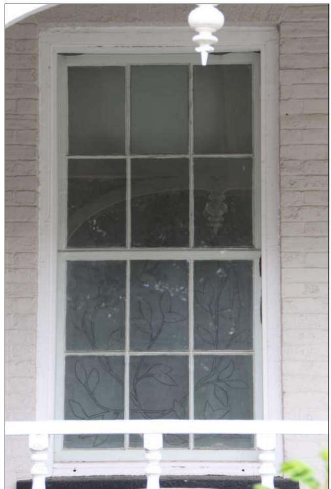
Figure 36 typical 6/6 double-hung sash window
