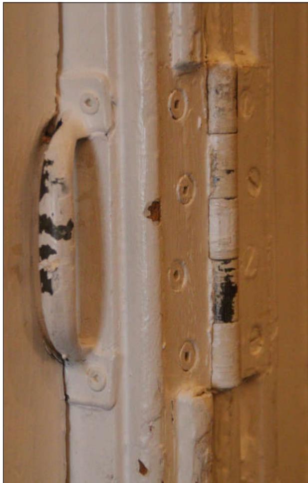
Figure 46 pocket door hinge & handle
