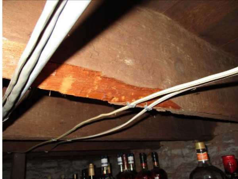
Figure 1: Deteriorated floor framing
