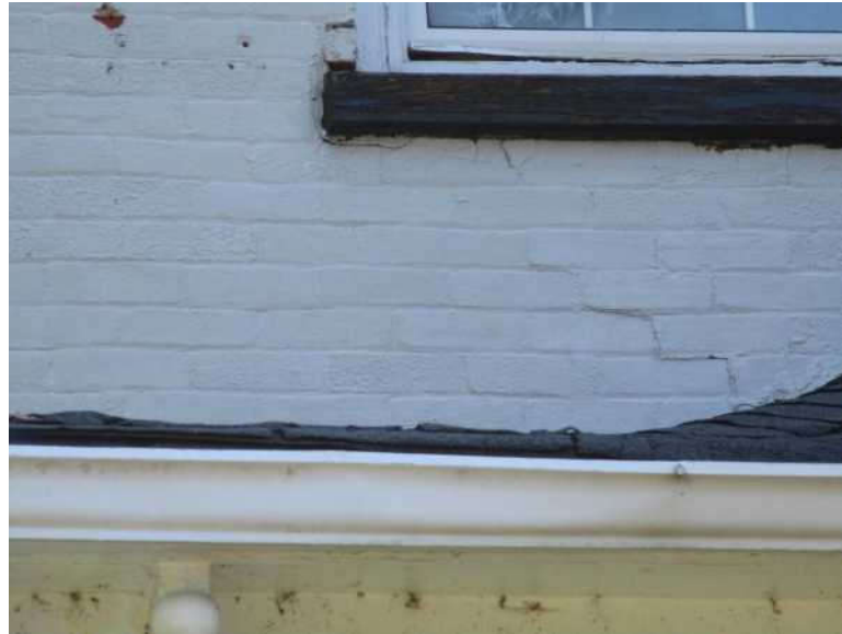
Figure 7: Step cracking below second storey window
