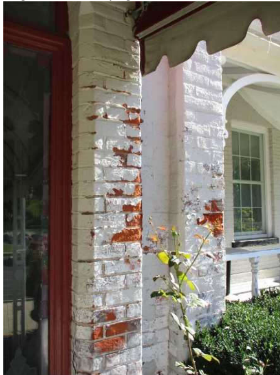
Figure 5: Deterioration on south side of entry canopy
