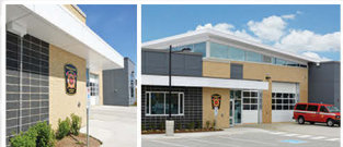
3 Fire Station 119 and Peel Regional Paramedic Satellite Station 6357 Airport Road
