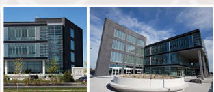
5 Kenaidan New Office Building 7080 Derrycrest Drive
