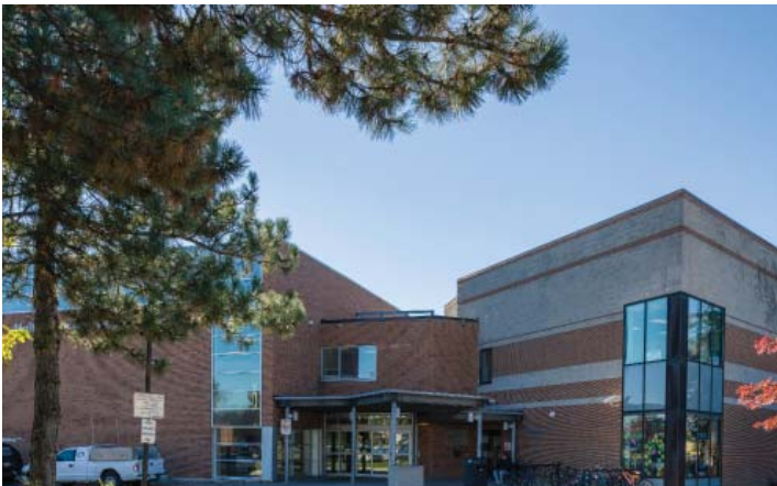
Malton Community Centre and Library
