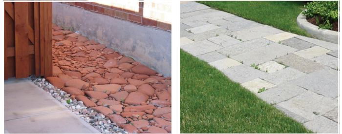
Fig. 41: Alternatives to asphalt and concrete promote on-site stormwater management.
