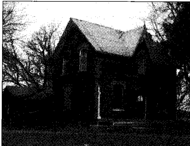
The historic McCauley House near the Erin Mills Town Centre is little more than a shell after fire gutted the building Sunday. Arson is suspected.
