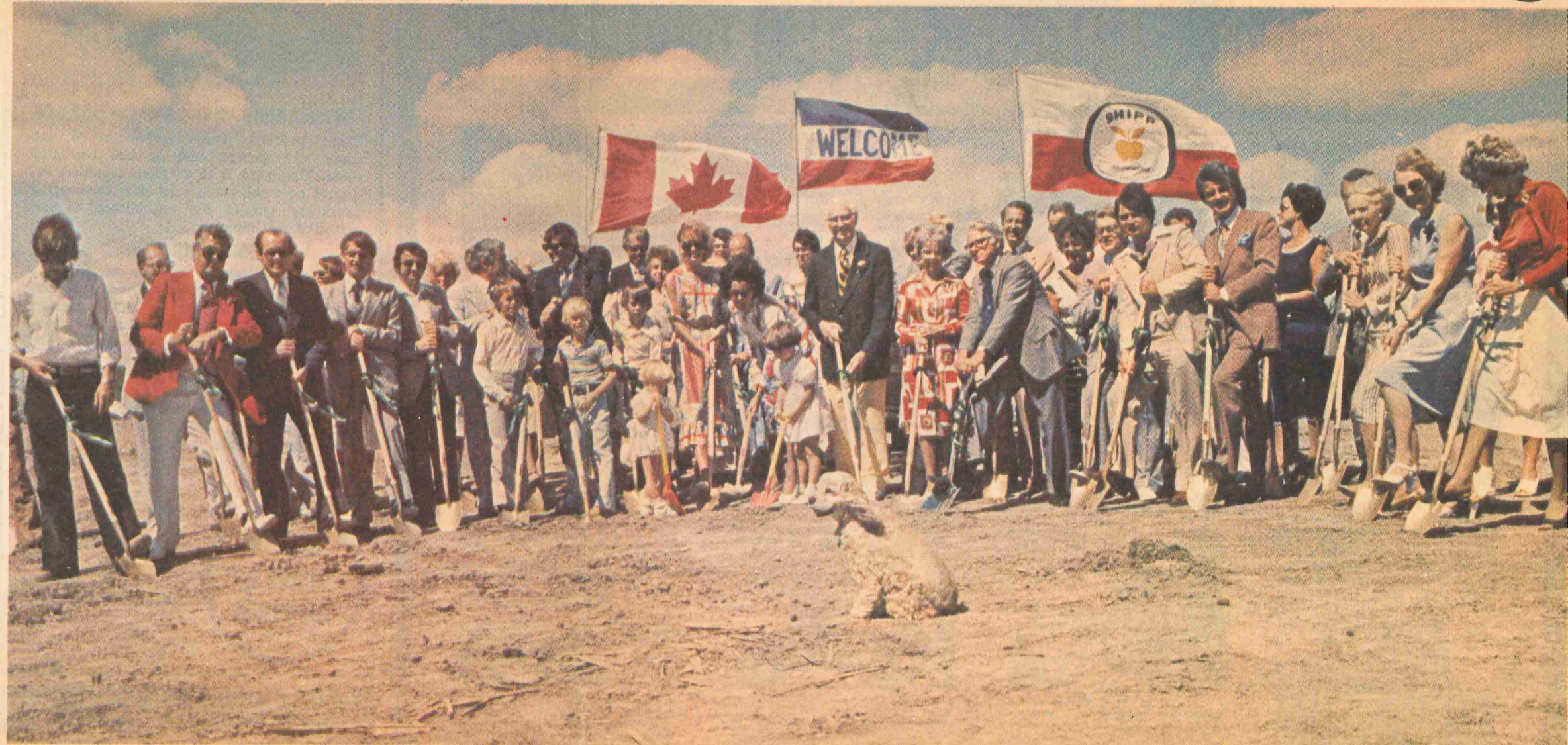
When the Shipp Corporation hosts a ground breaking, there's no fooling around. Everybody digs. Even the dog. Included among the workers last week were mayor Ron Searle, Shipp Corporation founder and chairman of the board Gordon S. Shipp and Enid Speck, wife of the late Bob Speck, the former mayor after whom Robert Speck Pkwy. was named. There were 55 diggers in all, to help commemorate the 55th anniversary of the founding of the Shipp Corporation.
