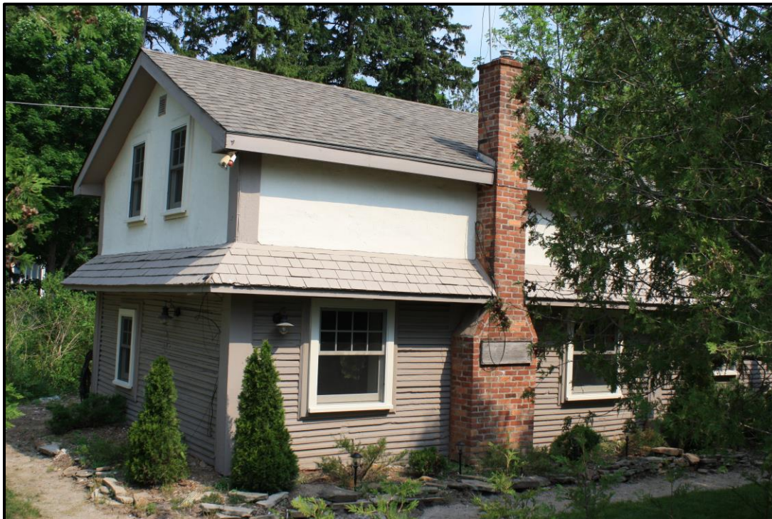
1101 Old Derry Road – Note the stacked plank construction on the lower half of the structure. The upper floor has been modified from the original structure.
