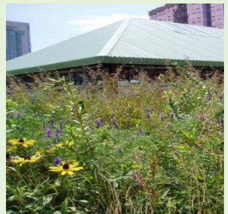
Figure B77 — Extensive Green Roof Above — Mountain Equipment Co-op
