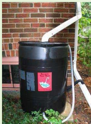
Figure B76 — Typical rain water barrel
