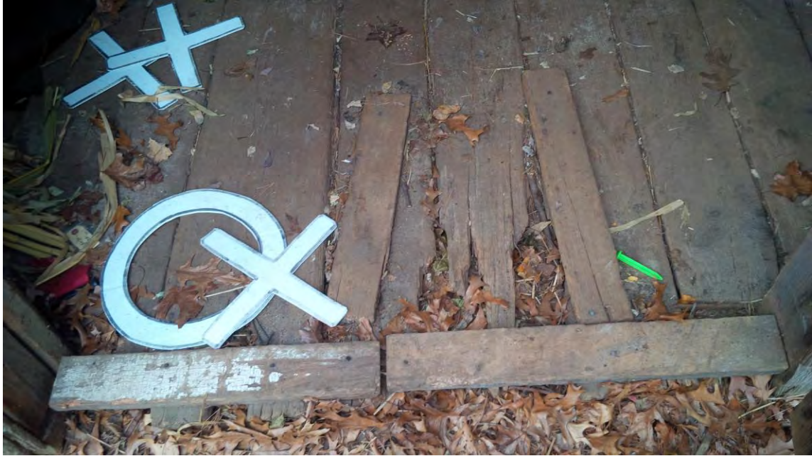
5.2.9. Typical example of deterioration and wear of Barn and Potting Shed floor boards.
