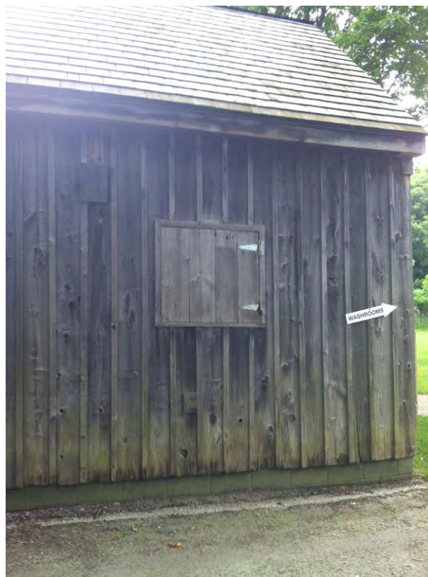
5.2.4. Barn – Detail elevation showing weathering of boards at base of exterior walls.
