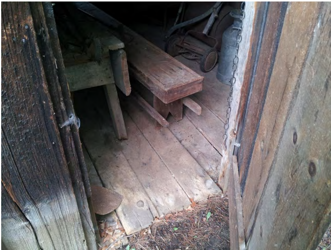
5.2.10. Typical example of deterioration and wear of Barn and Potting Shed floor boards.
