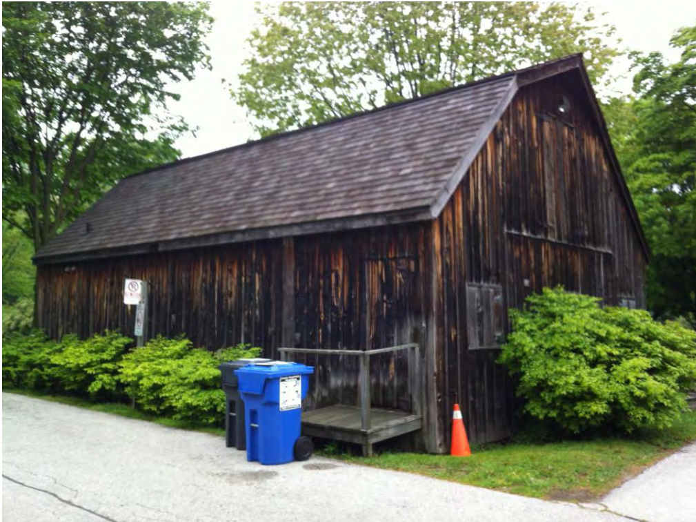
5.2.1. Barn – Elevation showing discoloration and uneven weathering.
