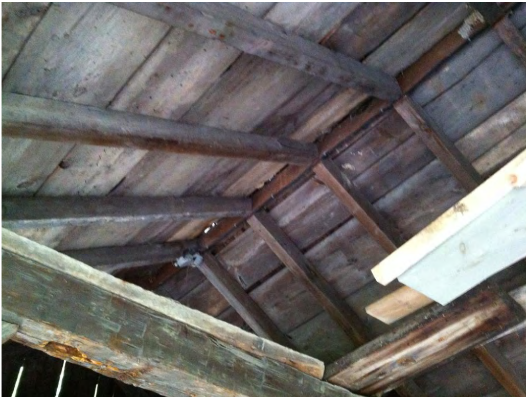
5.2.8. Shed – Interiors of shed showing existing wood framing conditions.
