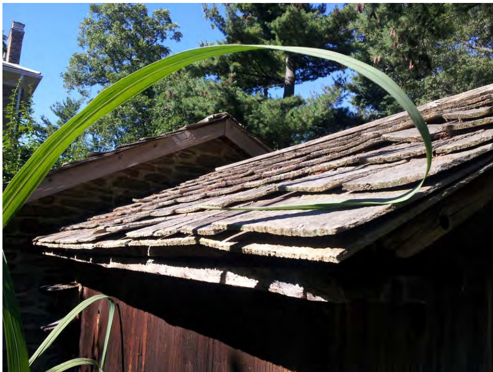
5.2.6. Dairy House – Sample of deterioration and weathering of cedar shingles and fascia boards.
