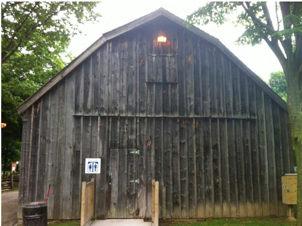
5.2.2. Barn – Elevation showing uneven weathering and separation of joints.
