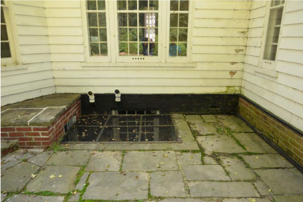
5.2.5. South Building Elevation – Sample of existing foundation wall and window well conditions.
