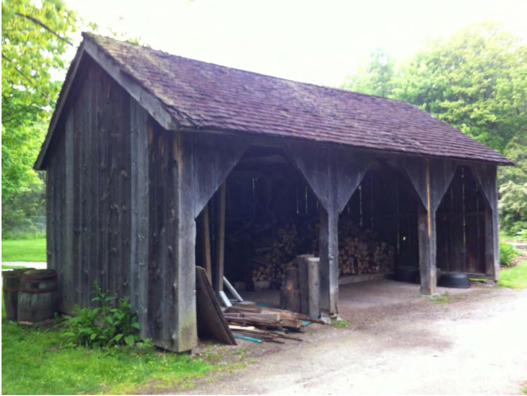
5.2.5. Shed – Elevation showing weathering of boards and on walls and columns and uneven discolouration.
