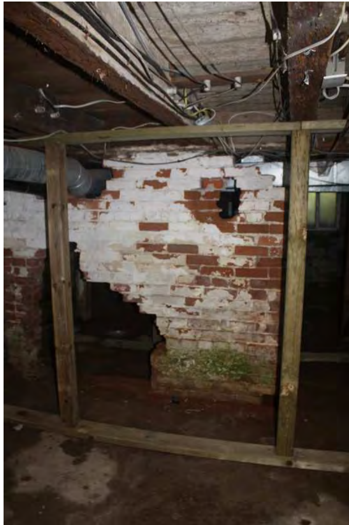
Figure 51 A gap in the interior basement wall of the original farmhouse and supporting timbers, 2013 (Photo by author.)
