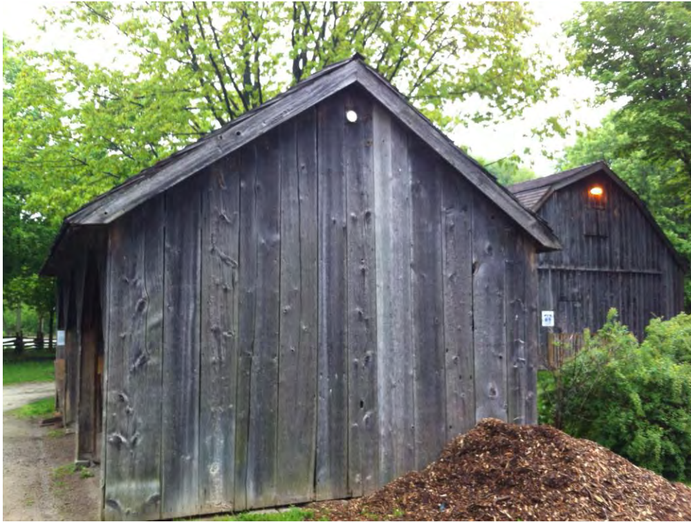
5.2.7. Shed – Elevation showing separation of boards and wear.
