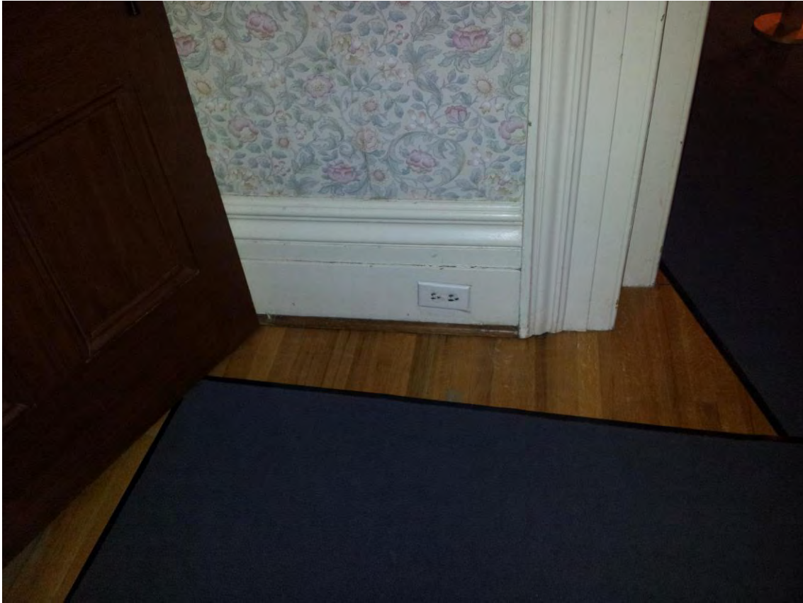
5.2.3. Main House – Sample of deterioration and wear of upper layer of wood floor finish.
