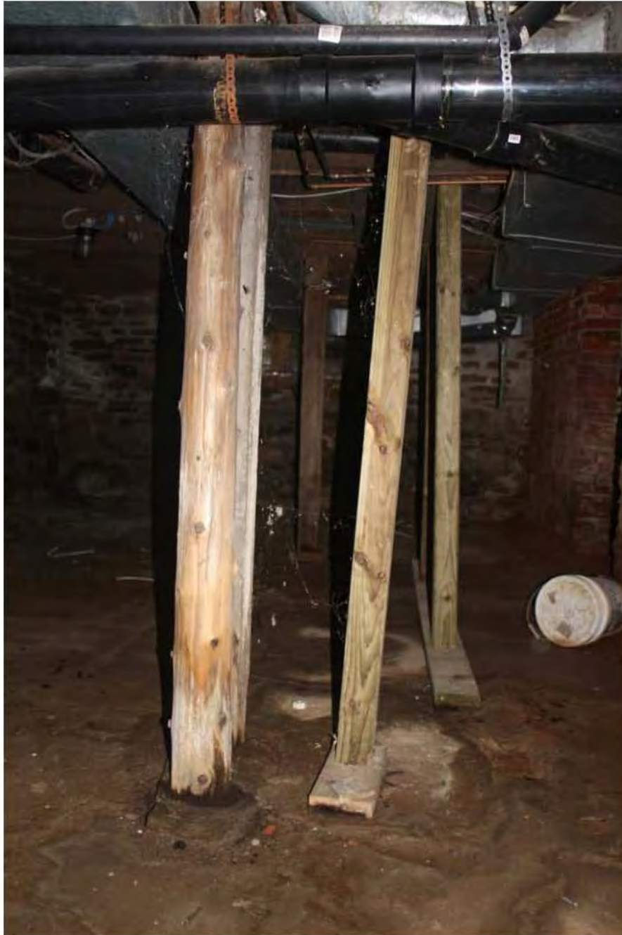
Figure 50 timber supports in the basement of the original farmhouse, 2013 (Photo by author.)
