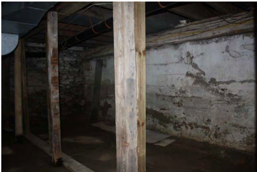
Figure 49 The basement of the addition, 2013. Timber had been inserted to support the structure (Photo by author.)
