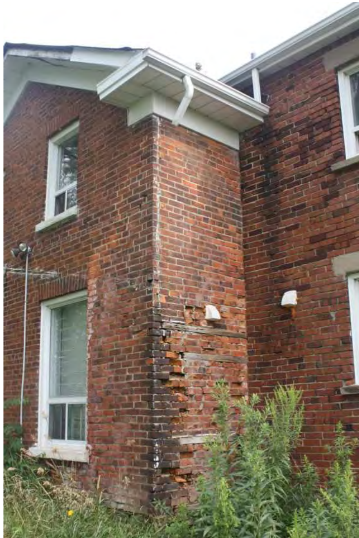
Figure 29 Deteriorating brickwork at the southwest corner of the original farmhouse, 2013 (Photo by author.)
