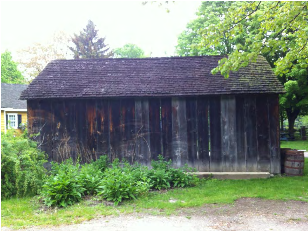
5.2.6. Shed – Elevation indicating uneven discolouration and separation of boards.
